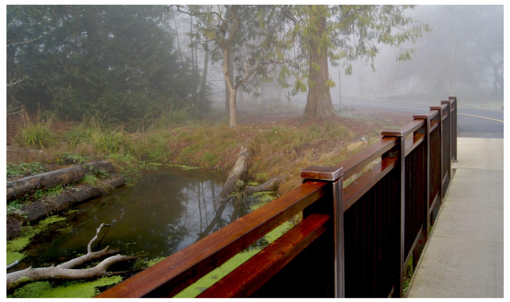
Although not certified under a rating system, sustainability drove materials selections. Using weathering steel for bridges and railings instead of standard galvanized or painted steel prevented zinc and paint from entering the stream. Irrigation piping was HDPE instead of PVC.
