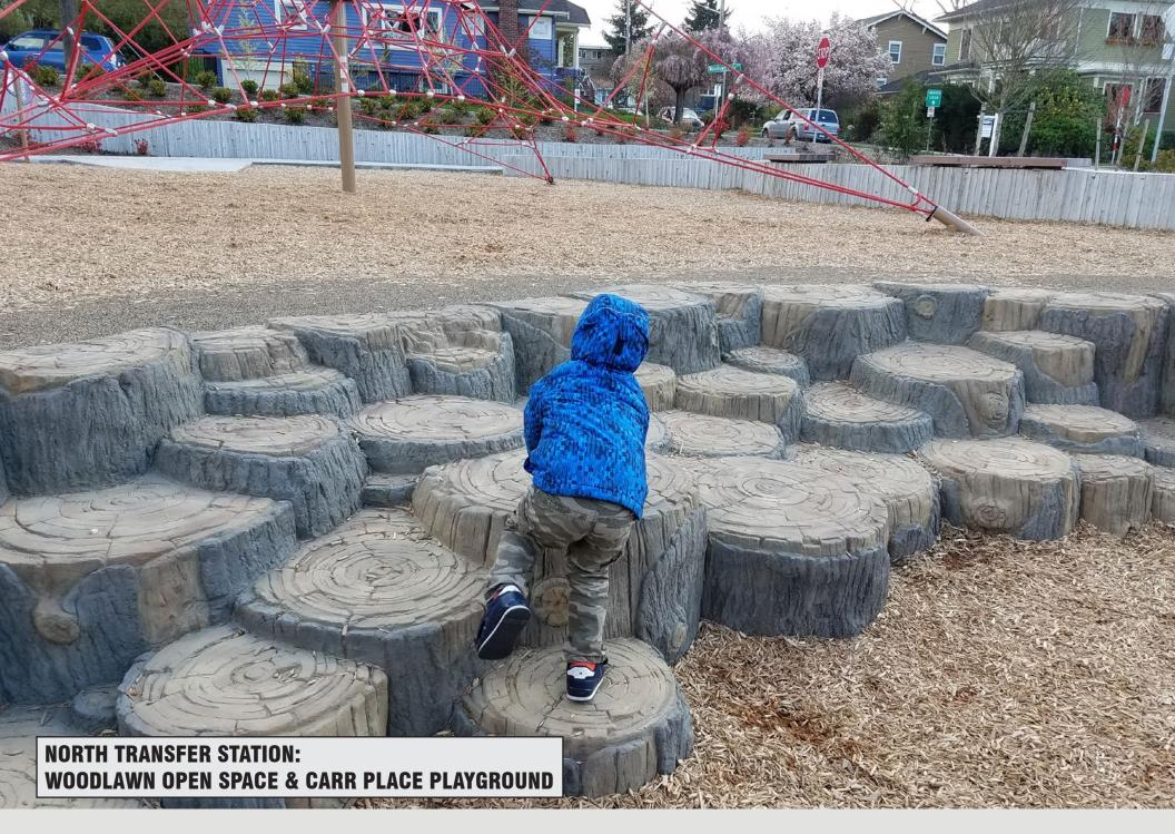
Custom-designed, glass fiber reinforced concrete "log steppers" transform retaining walls into fun and challenging climbing features that blend with the natural features of the playground.
