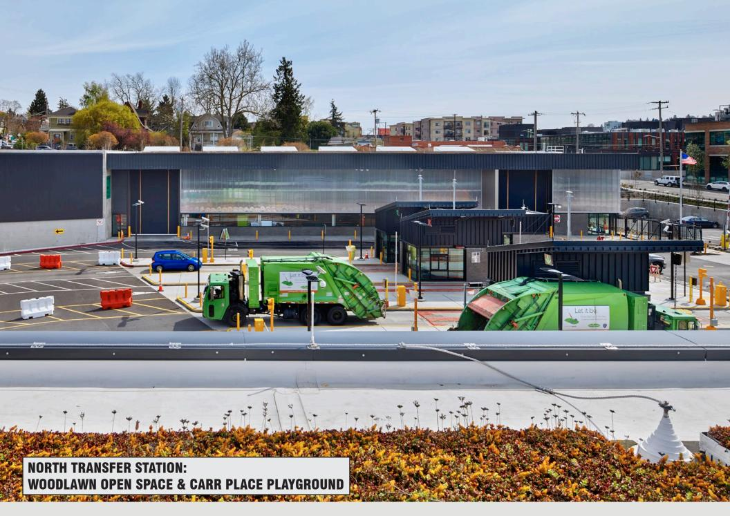
The new facility reduces congestion on neighboring streets by accommodating over 50 vehicles on site, and handling 400 tons of material a day, with an expansion capacity of 750 tons as population growth in the city continues.
