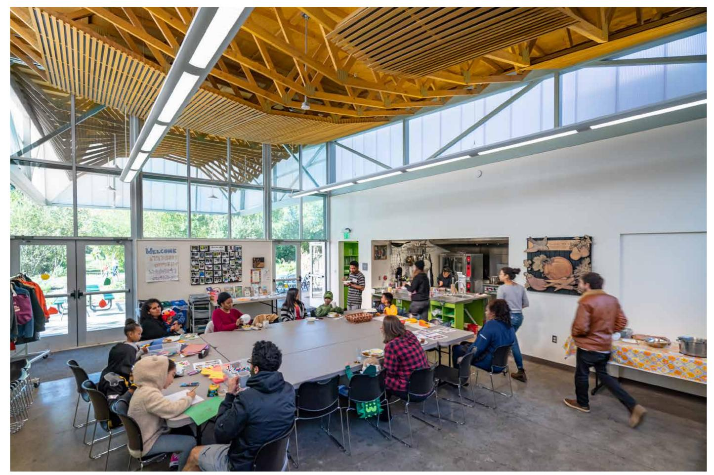
Large and flexible in design, the building's easily maintained, polished concrete floor extends into the terrace beyond. The truss system maximizes open space inexpensively while translucent panels provide ample daylight with a nod to a common greenhouse material.
