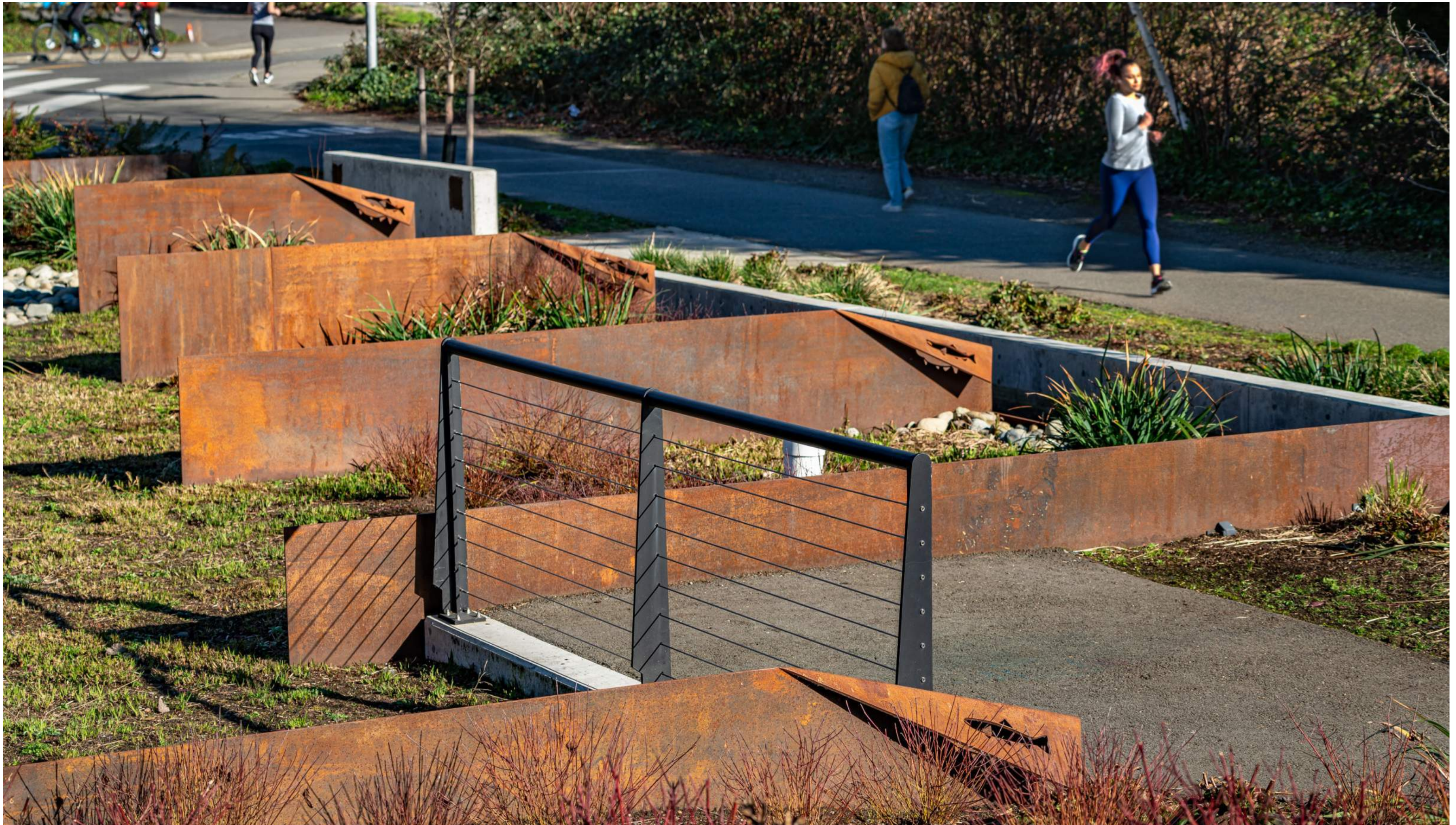
THE SWALES RAISE AWARENESS TO THE REGION'S STORMWATER QUALITY ISSUES BY ENGAGING THE ONE MILLION PEOPLE THAT USE THE ADJACENT BURKE-GILMAN TRAIL ANNUALLY.
