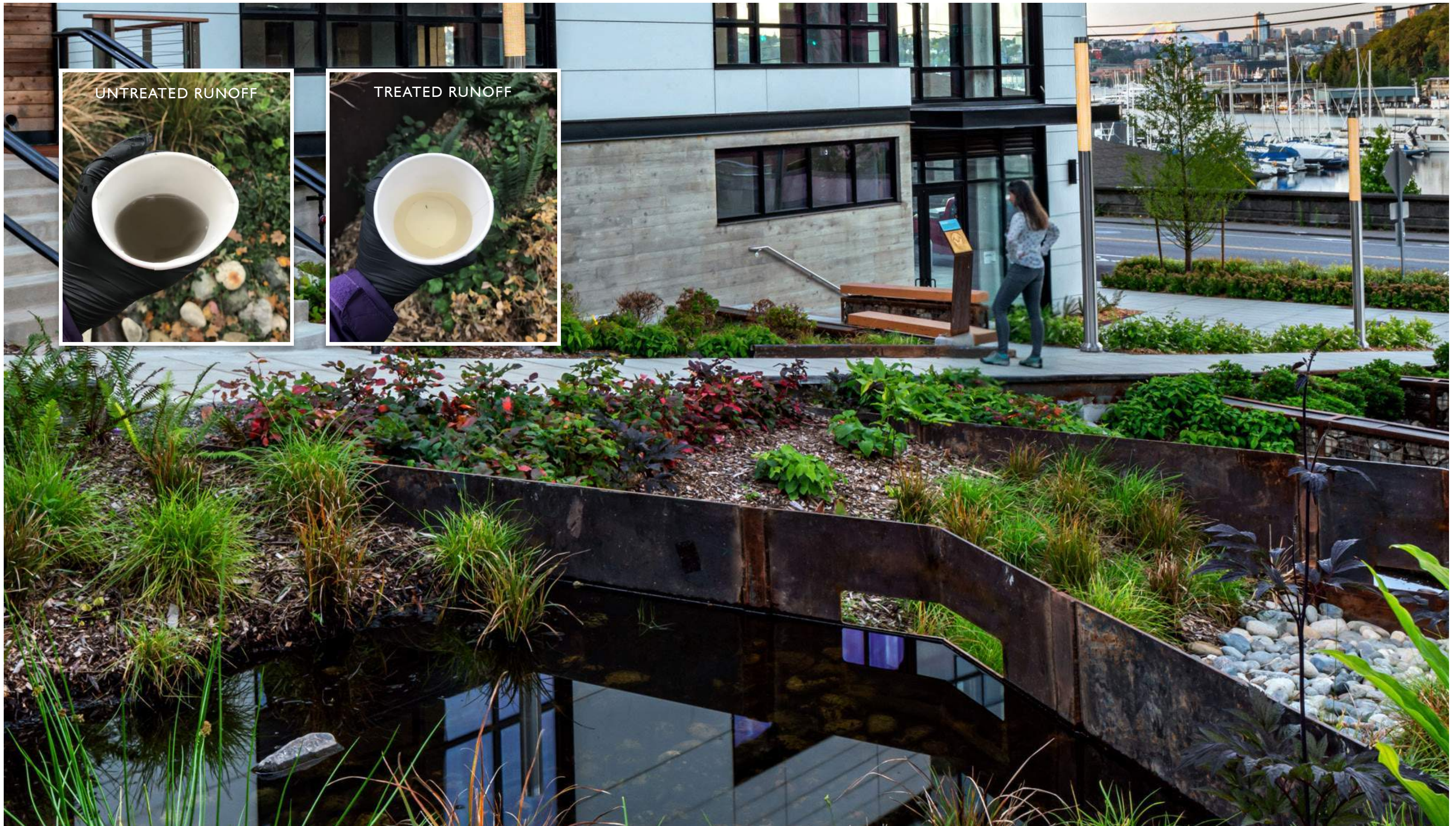
MEASURABLE TESTING CONFIRMS THAT AS THE WATER FILTERS DOWN THE SWALES IT BECOMES CLEANER AND LESS CONTAMINATED.
