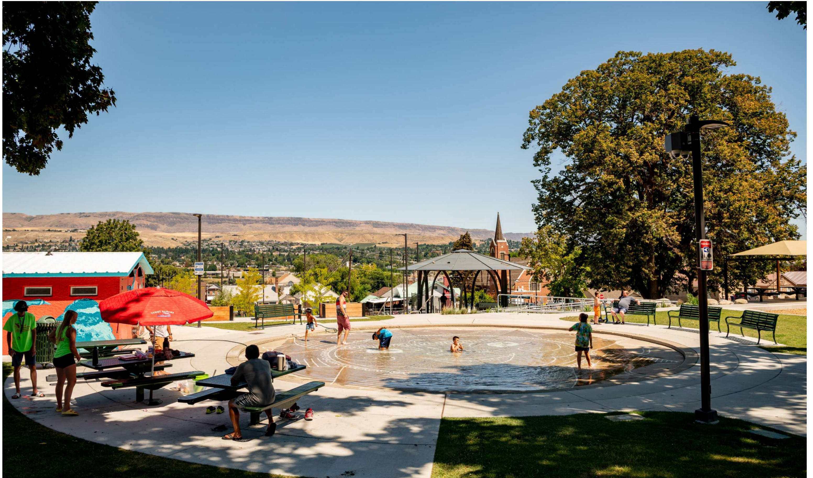
A new loop pathway, picnic area and restroom building revitalize the area around an existing wading pool, providing amenities for all ages. The story of migration continues in a mural on the new building.
