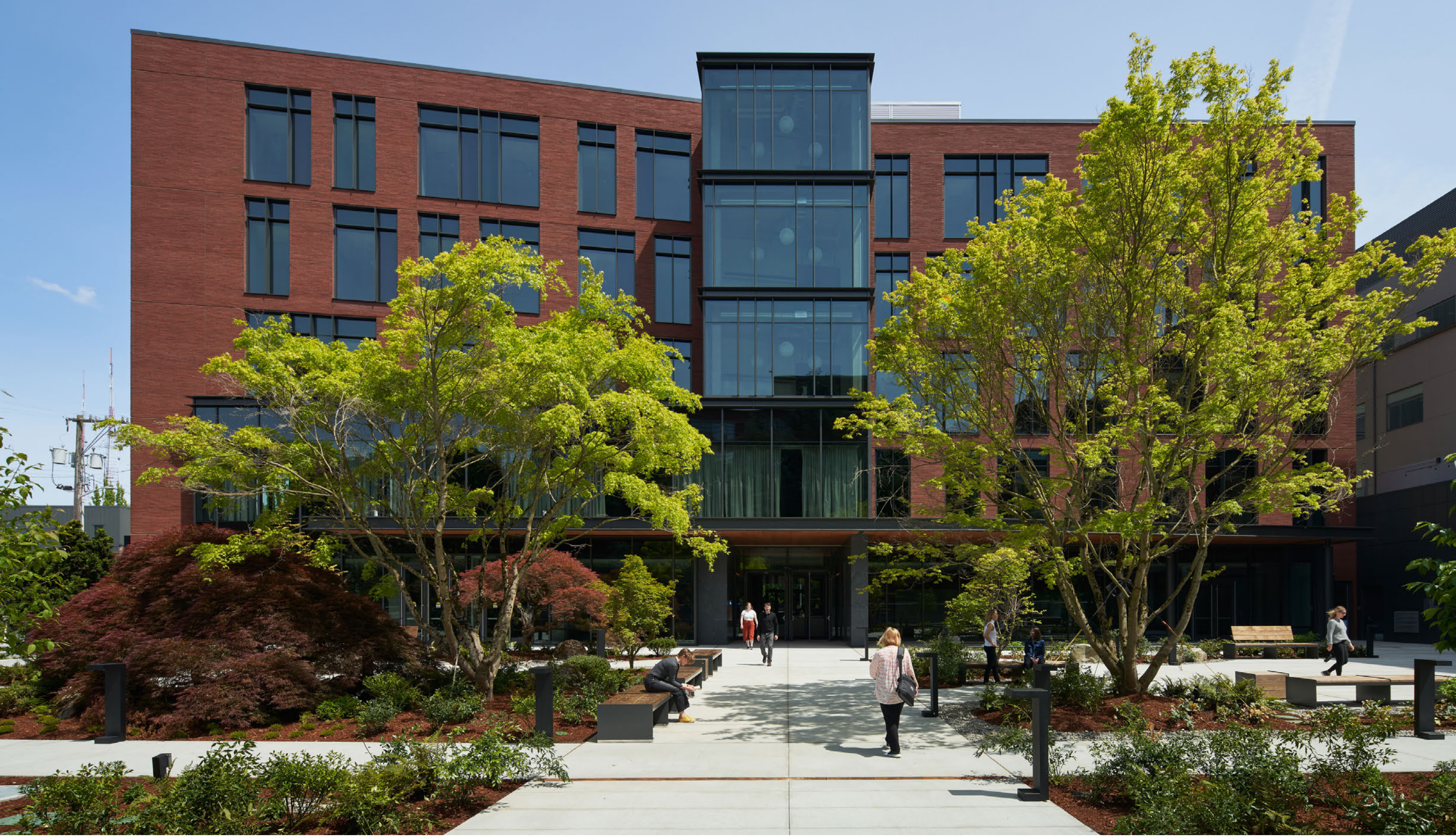
The west side is separated by a wide mid-block connector, dotted with custom benches to provide places to rest. The southern courtyard is more open, providing a large, flexible open space for events and class experiments.
