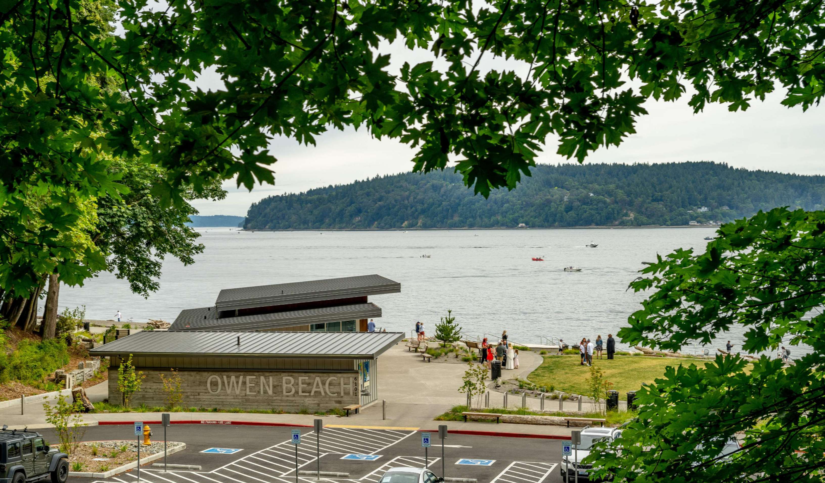
Holding the new shelterhouse and restroom facilities close to the hillside kept the sweeping views of Puget Sound at the focus of the reconfigured arrival sequence.
