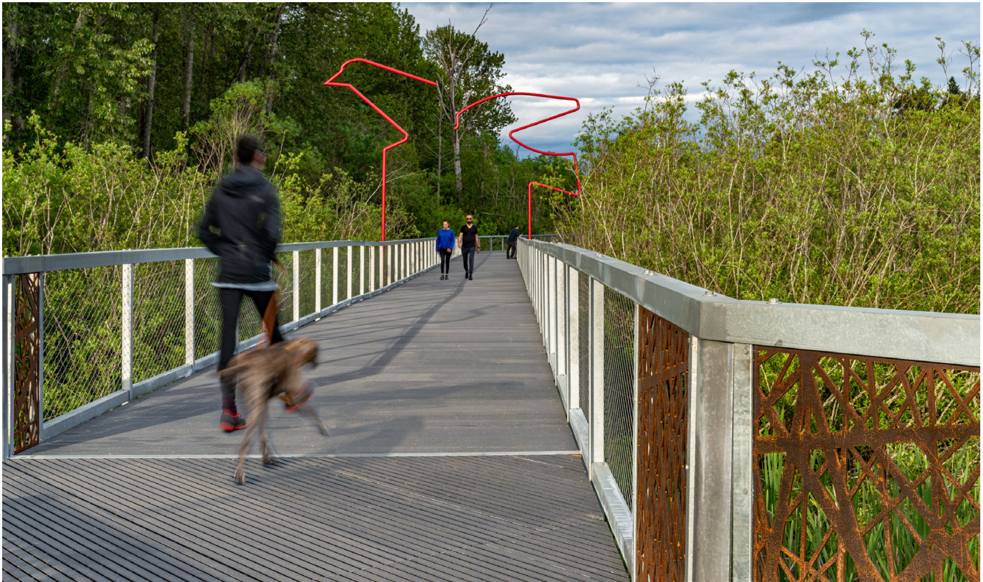
The boardwalk connects people to nature and is a primary connector between a vibrant new community and a regional multimodal trail. Widened during design to accommodate a range of users, the boardwalk's angular geometry slows cyclists and minimizes wetland impacts.
