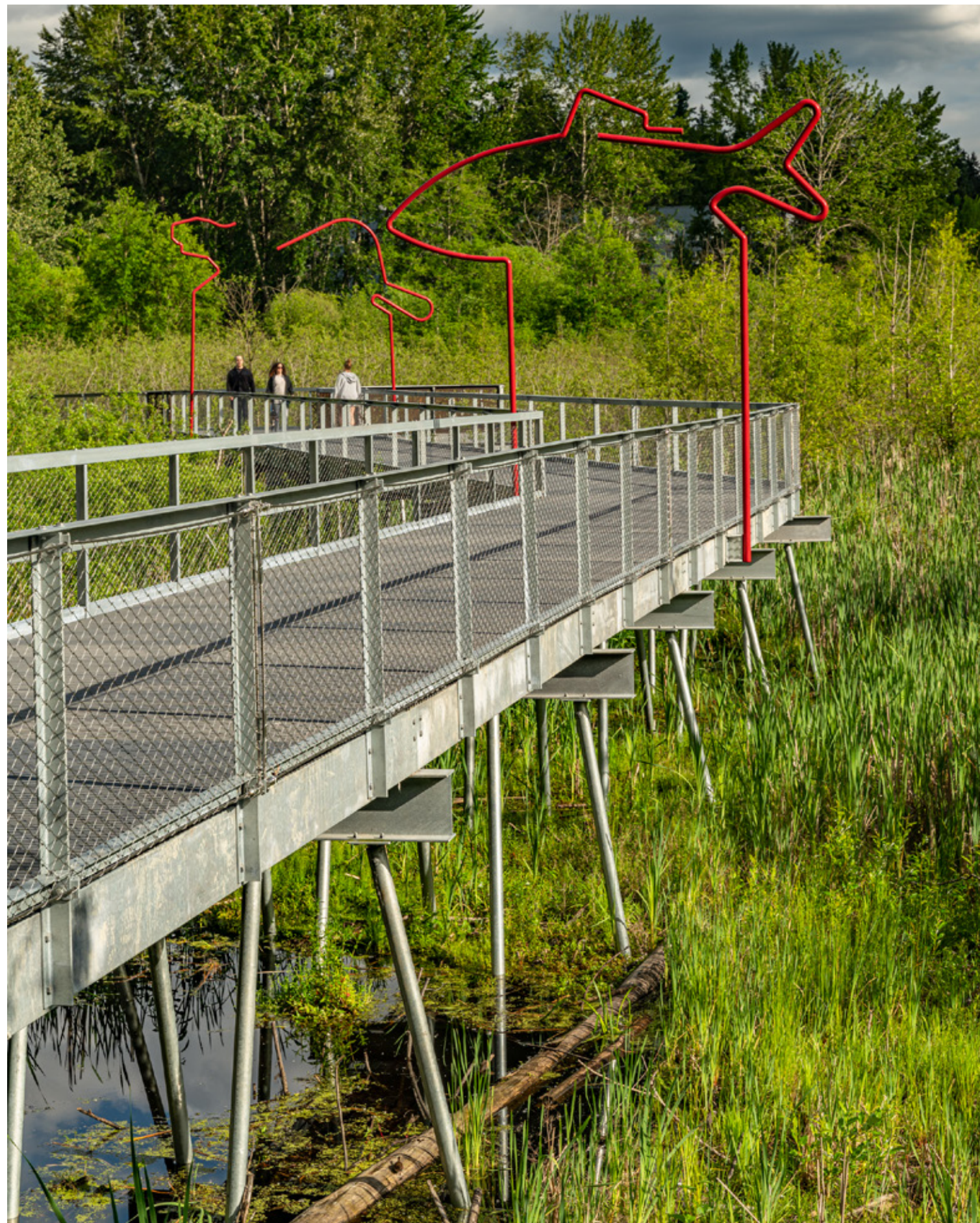
To minimize impacting the wetlands, work platforms and construction methods avoided digging or major ground disturbance. The structure is engineered to maximize spans between beams and rises above vegetation. Vegetation that was cut quickly re-established after construction was complete.
