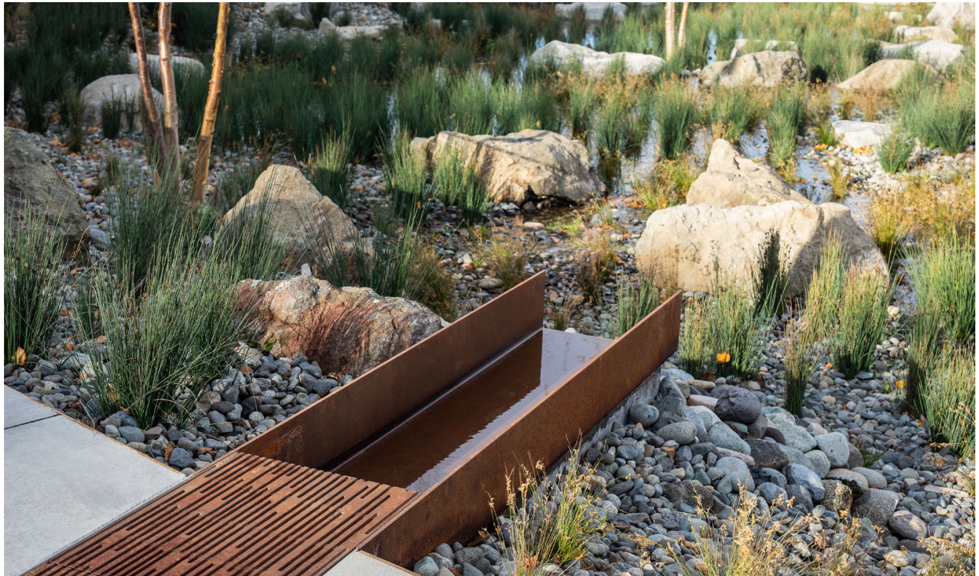
Weathering steel runnels inscribed with quotes contrast with the unpigmented concrete. Weathering steel, in lieu of other metals, is deemed safe for fish by limiting zinc in the watershed. Revealing and celebrating stormwater builds appreciation and understanding of stormwater management.
