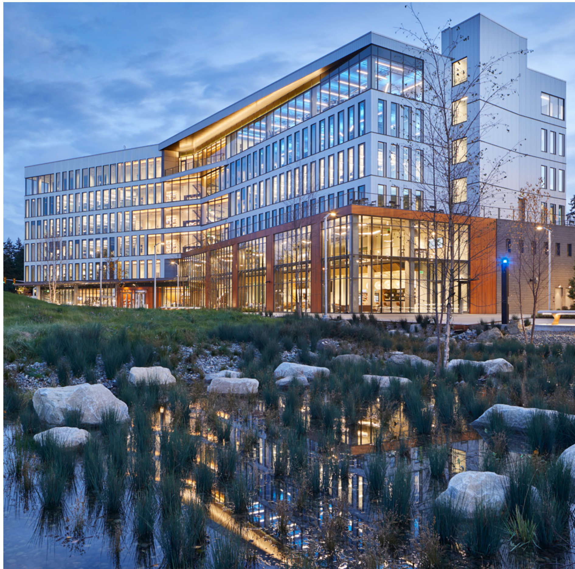
Water is a key tenet to the concept and story of place. Designed to handle five future buildings and associated paved areas, the rain garden slowly infiltrates to an underground detention chamber reducing impact to the city's stormwater system.
