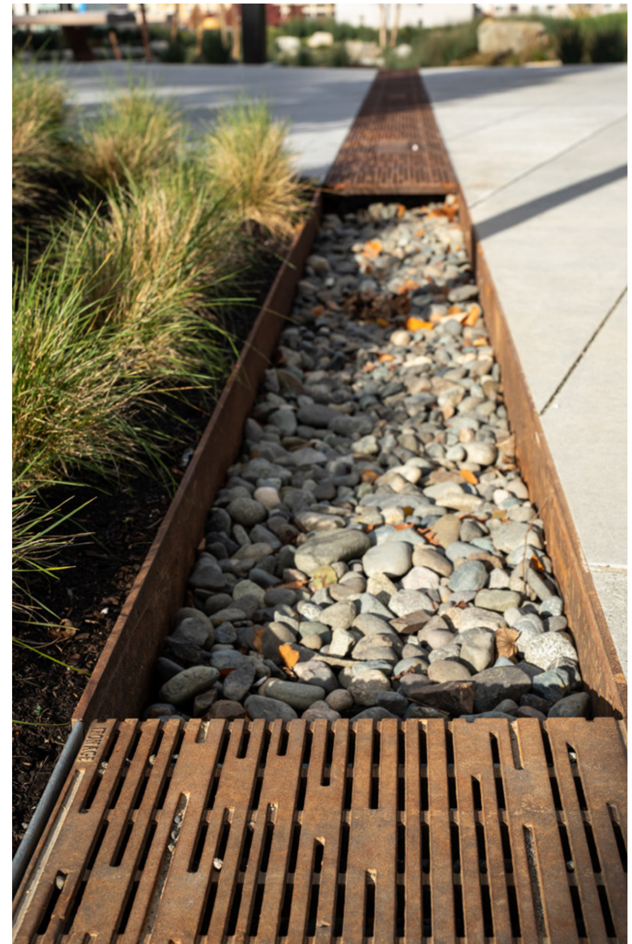
Water is a key tenet to the concept and story of place. Designed to handle five future buildings and associated paved areas, the rain garden slowly infiltrates to an underground detention chamber reducing impact to the city's stormwater system.
