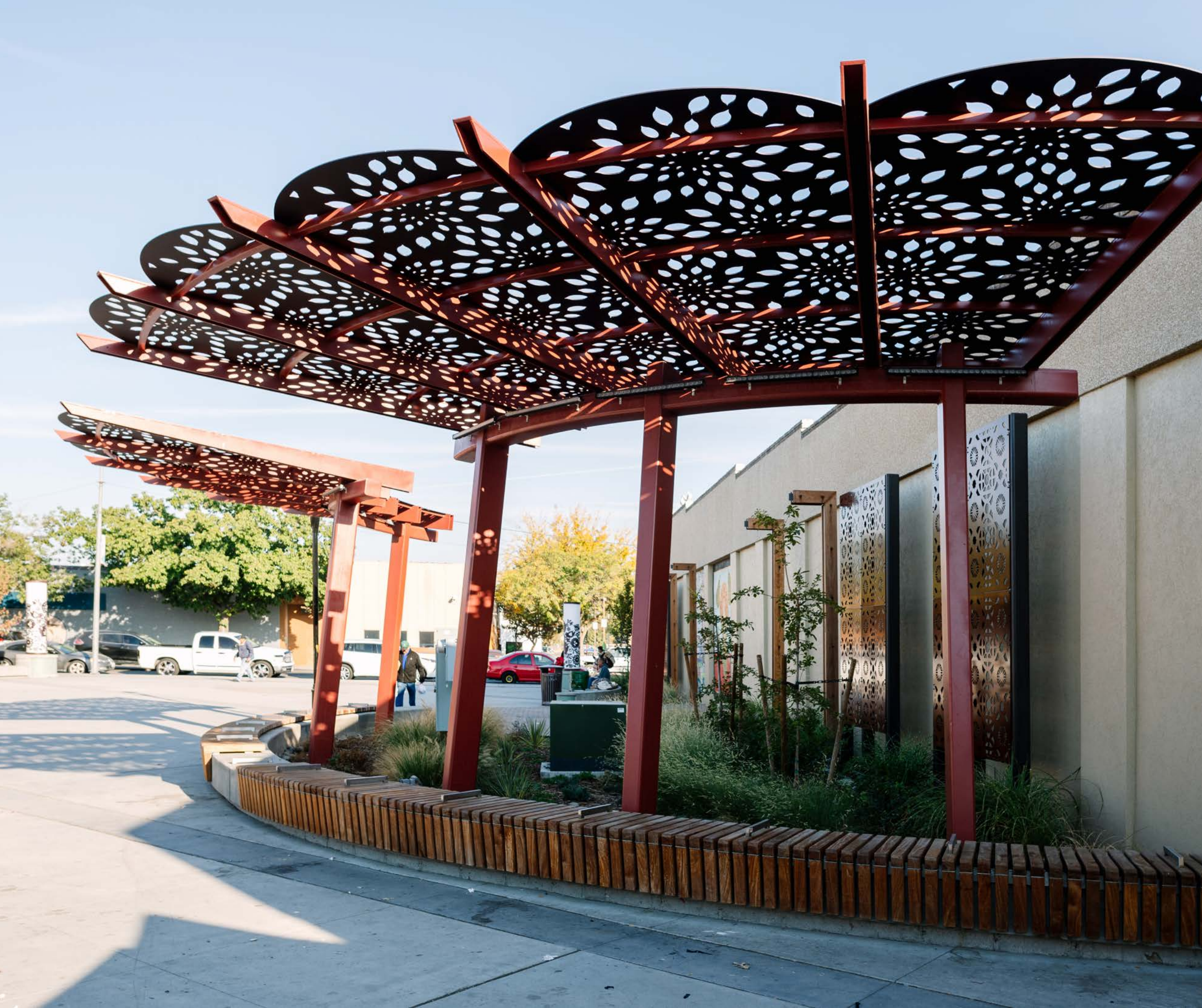
Custom shade structures provide instant shade on site where existing trees weren't able to be retained. The papel picado inspired pattern was used to provide a "leafy" shade canopy.
