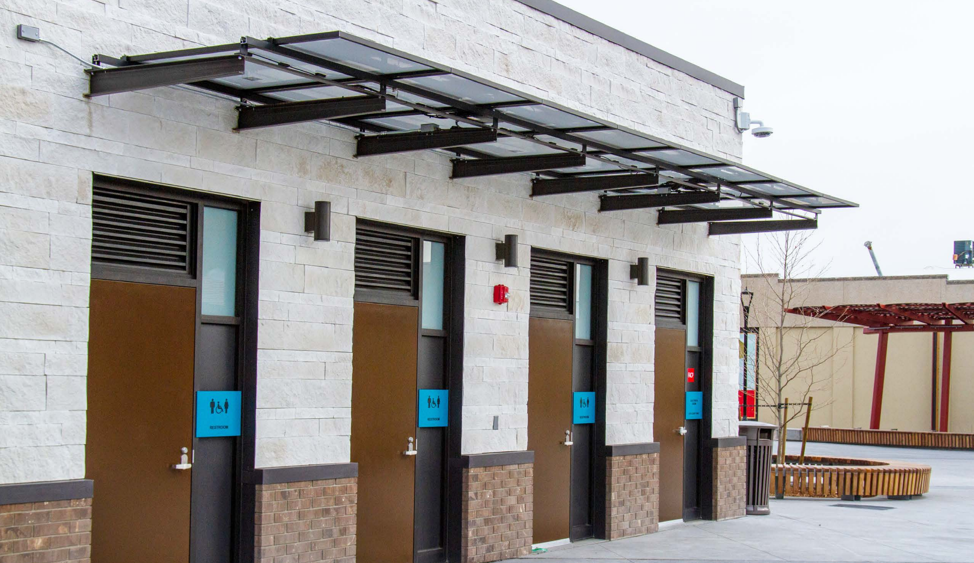
The new restroom building provides accessible, gender neutral restrooms with locking mechanisms, easy for City staff to manage. On-site storage allows for easy maintenance of the plaza. Solar panels are attached to the canopy to power the building.
