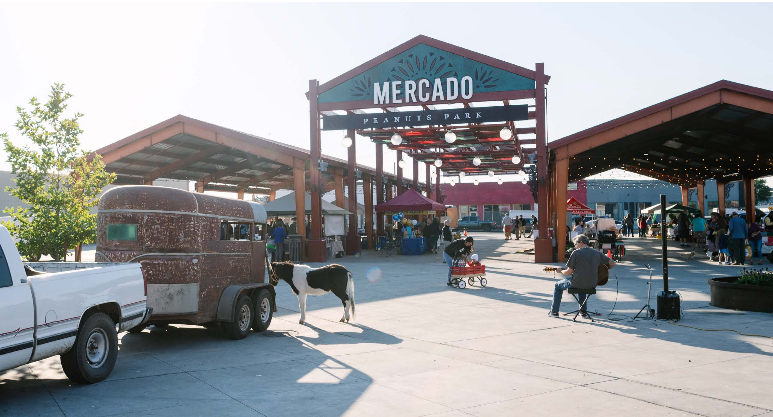
The reinforced concrete pavement allows vendors to drive on-site for easy setup/breakdown. The open layout, with carefully placed seating nodes, allows for a variety of activation opportunities such as live music, food trucks, or even pony rides!
