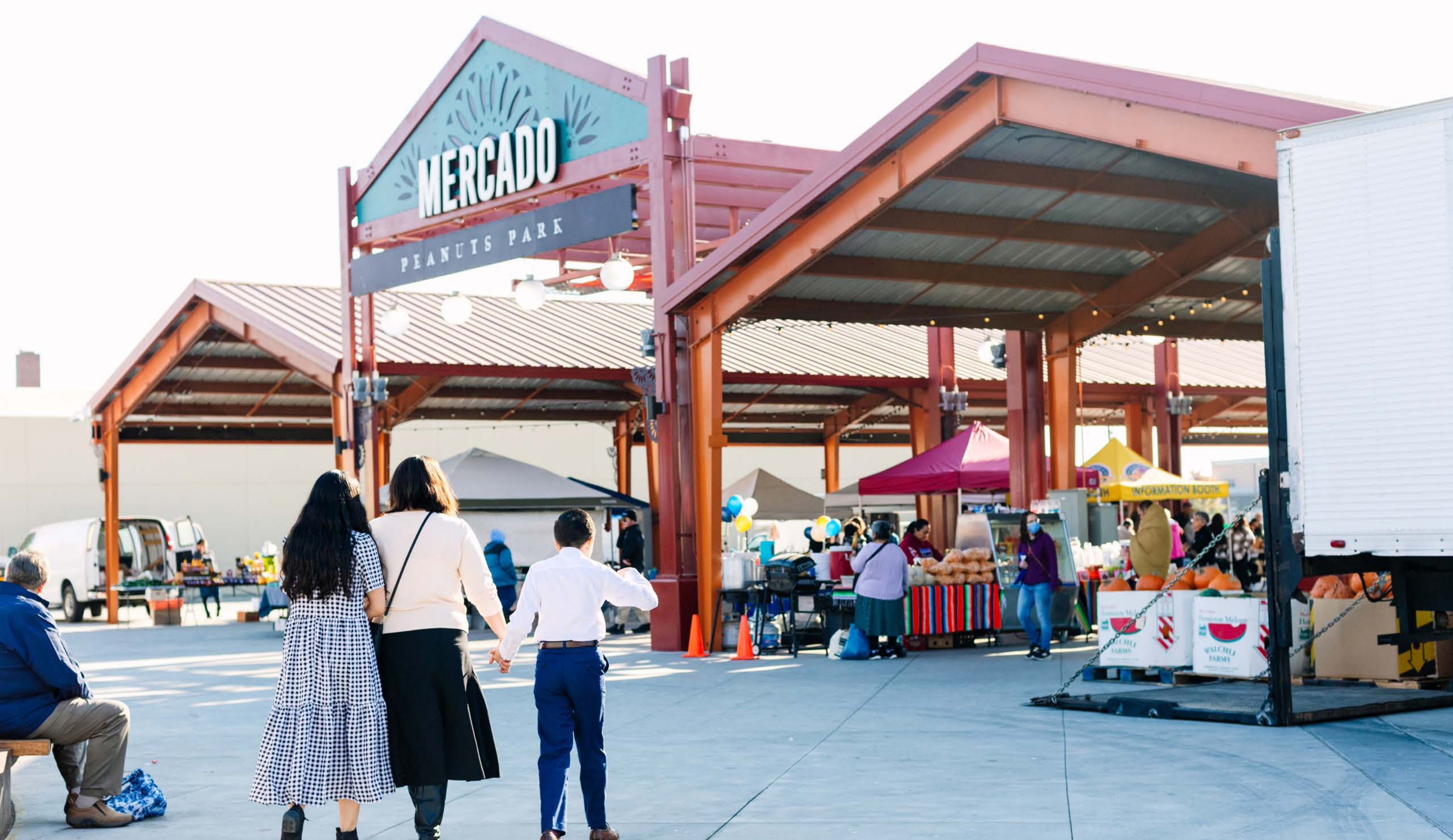
The new center structure “Gran Pasillo”, flanked by the refurbished pavilions house the weekly Farmers Market. These structures anchor the plaza providing a flex-use shelter for community events throughout the year, both large and small.
