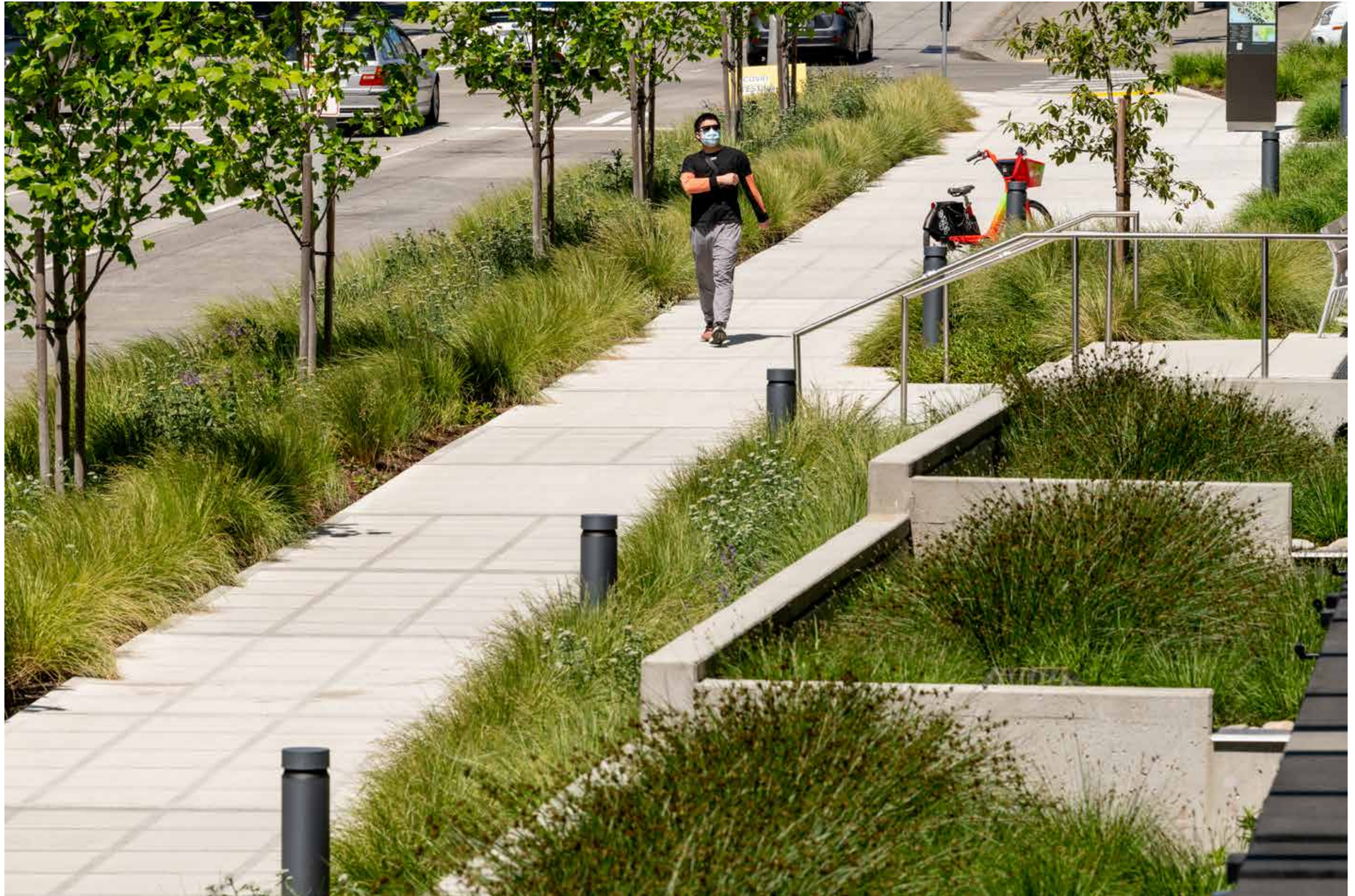
Stepped bioretention planters celebrate stormwater adjacent to the Center's interior gallery and provide interest to passing pedestrians. All pavement runoff is directed either into these structured bioretention facilities or to graded facilities along the project's interior lanes.
