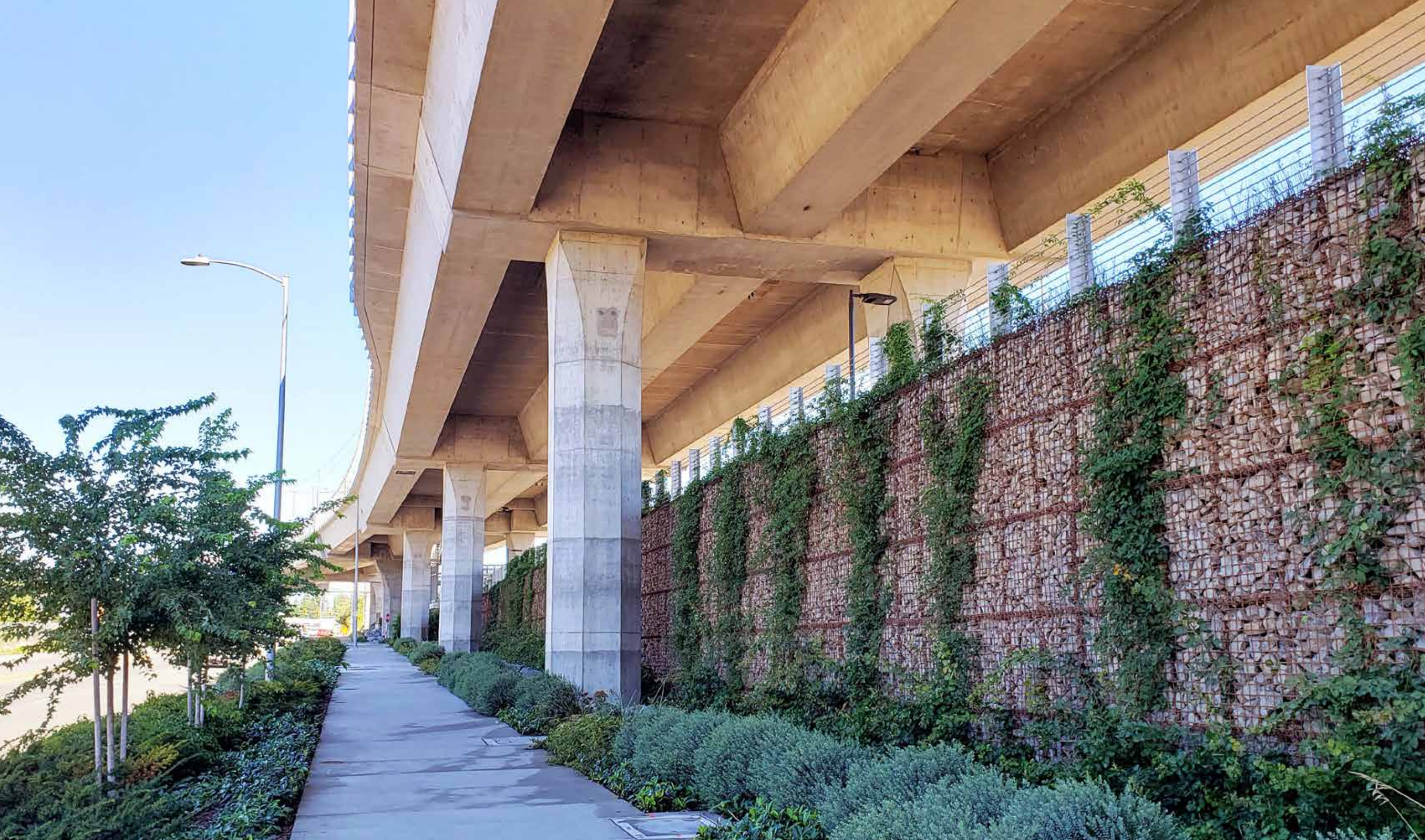
Trees, shrubs, and vines soften the pedestrian experience and place the guideway into context.
