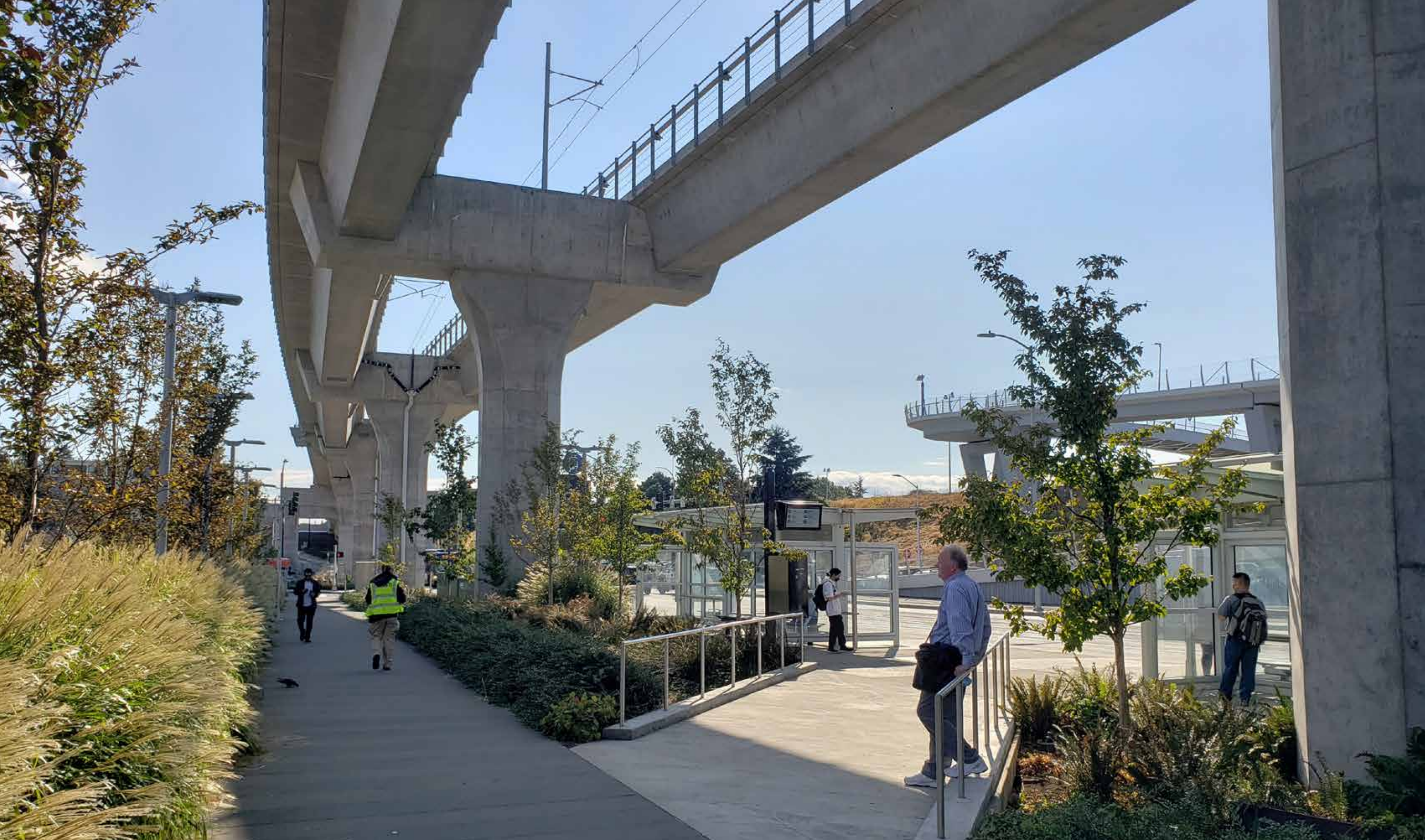
Bridges span the stormwater retention areas that match the scale of the guideway infrastructure. The generous pathways provide ample space for peak traffic, while also feeling protected and allowing people to stop and look over the rain gardens.
