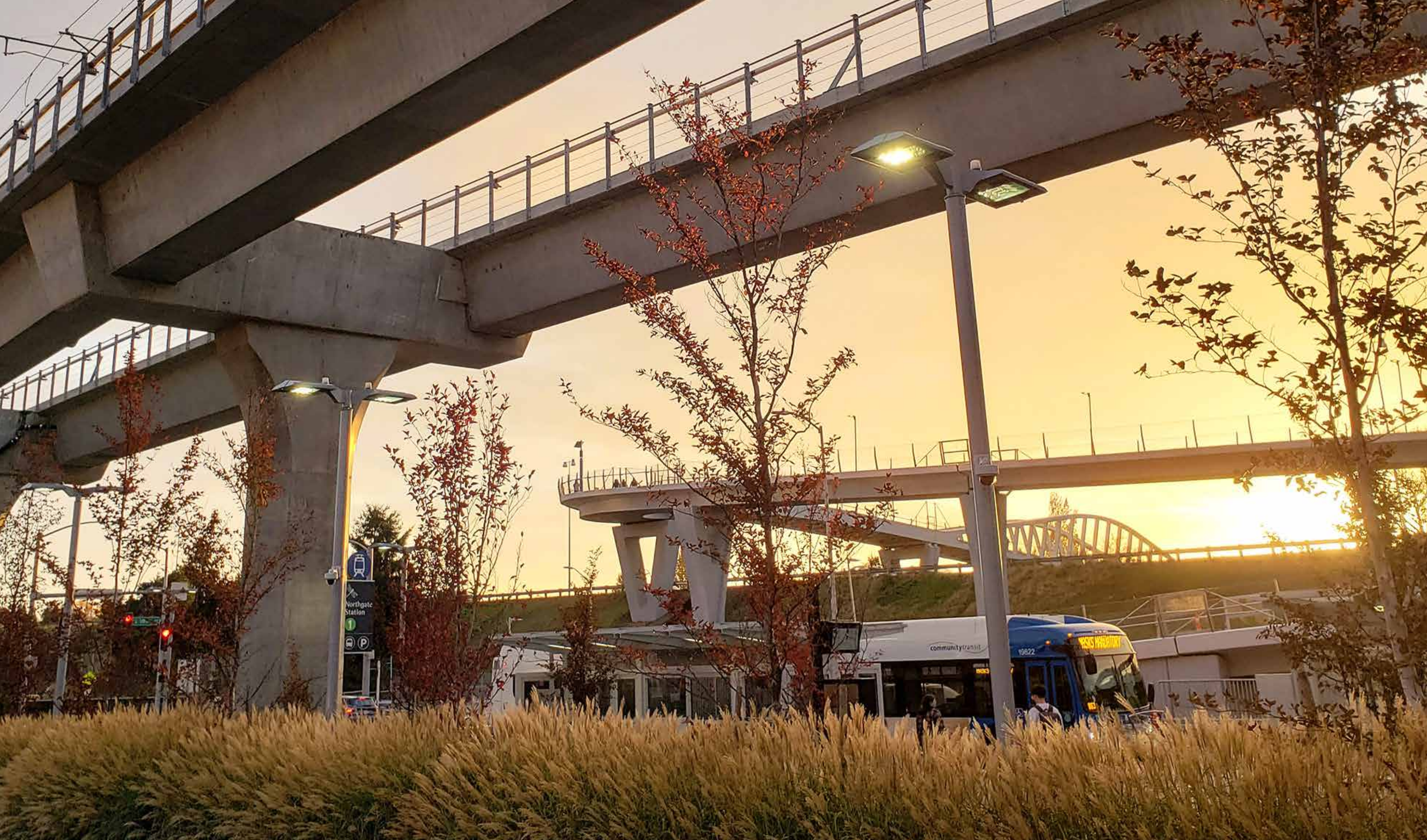
The late afternoon light turns the transit guideways above into a sundial, with shadows marking the passing of time as riders come and go. The dense grasses blowing in the breeze gives some life along the central corridor and evergreen vegetation covering the warm colored gabion walls root the station in this place.
