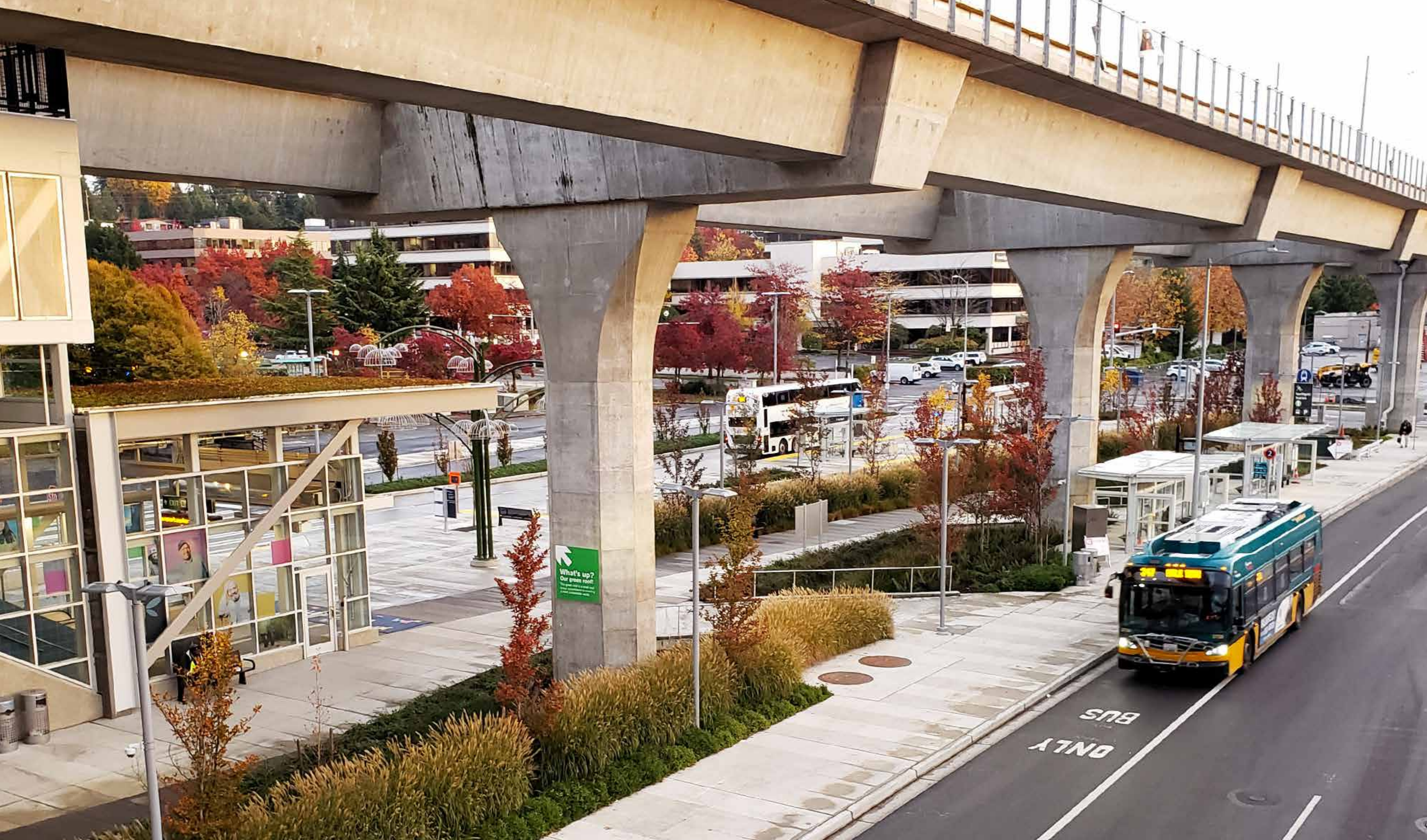
The overhead train platform is connected to the bus loops below. The scale of the stormwater and other planting areas matches the scale of the overhead infrastructure, harmonizing the two and balancing the visual weight of the systems. A green roof reduces the urban heat island effect and provides another layer of vegetation between the guideway and the street.
