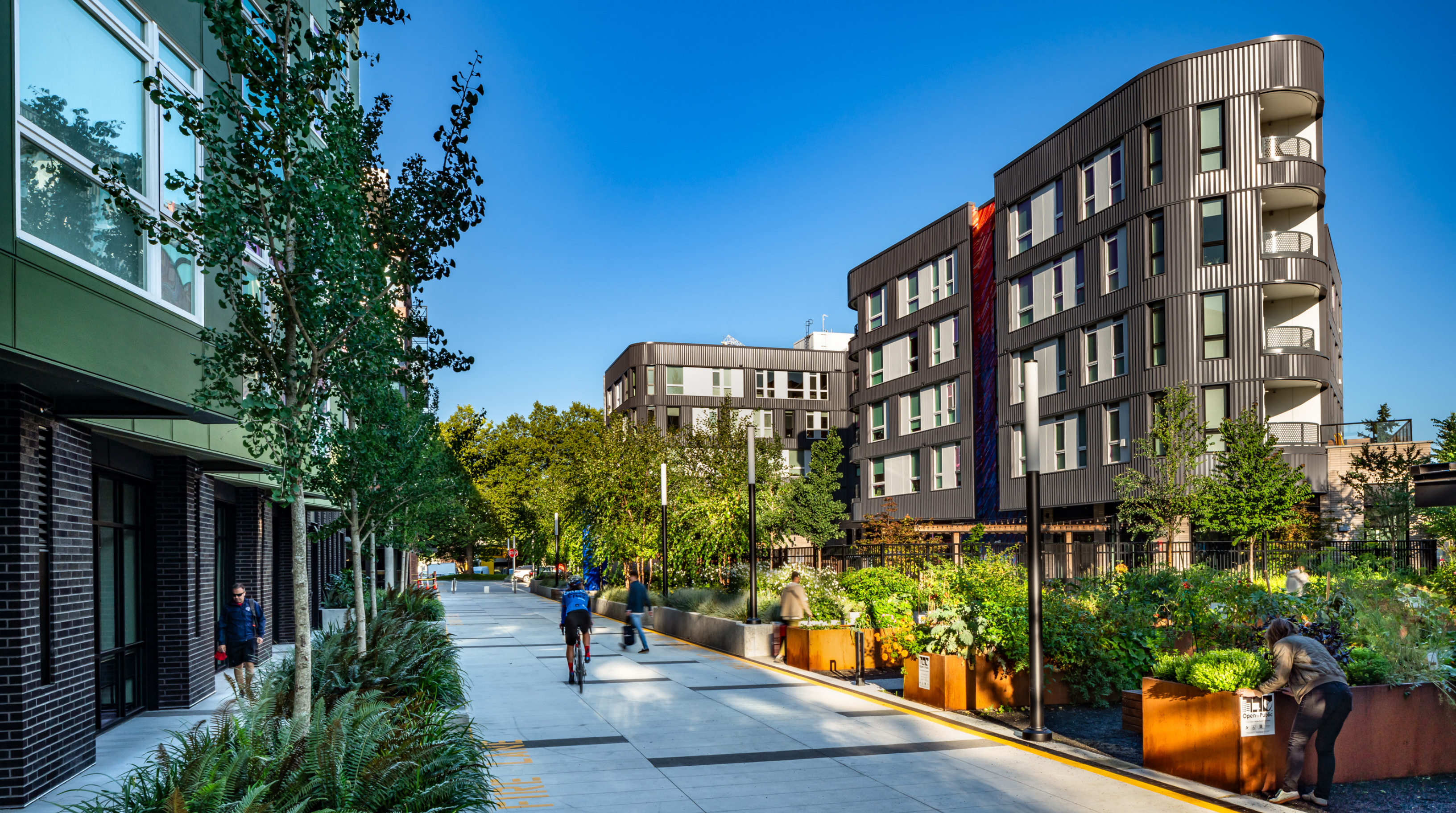
The popular east-west promenade creates a mixing environment for cyclists, pedestrians, residents and gardeners alike.
