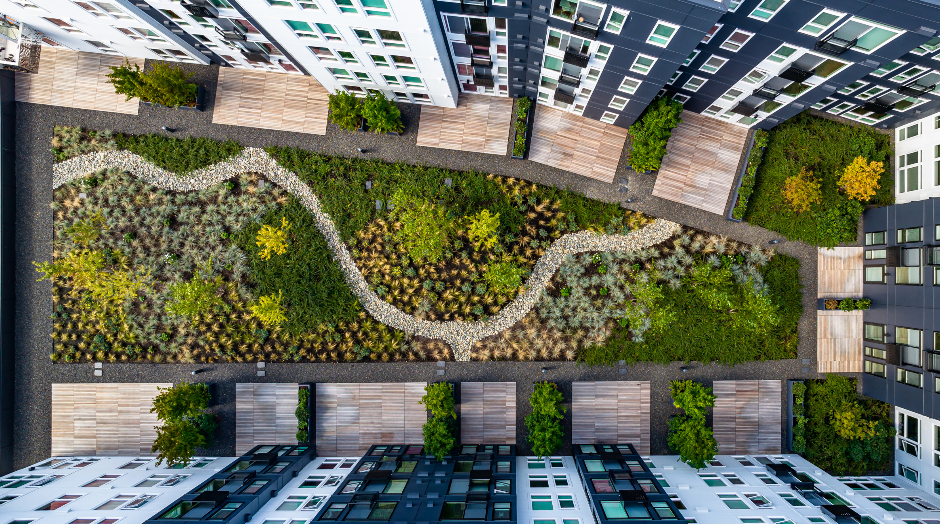
The undulating planting design of grasses, native trees and decorative cobble is revealed in the view of the second-story courtyard from the roof deck and units above.
