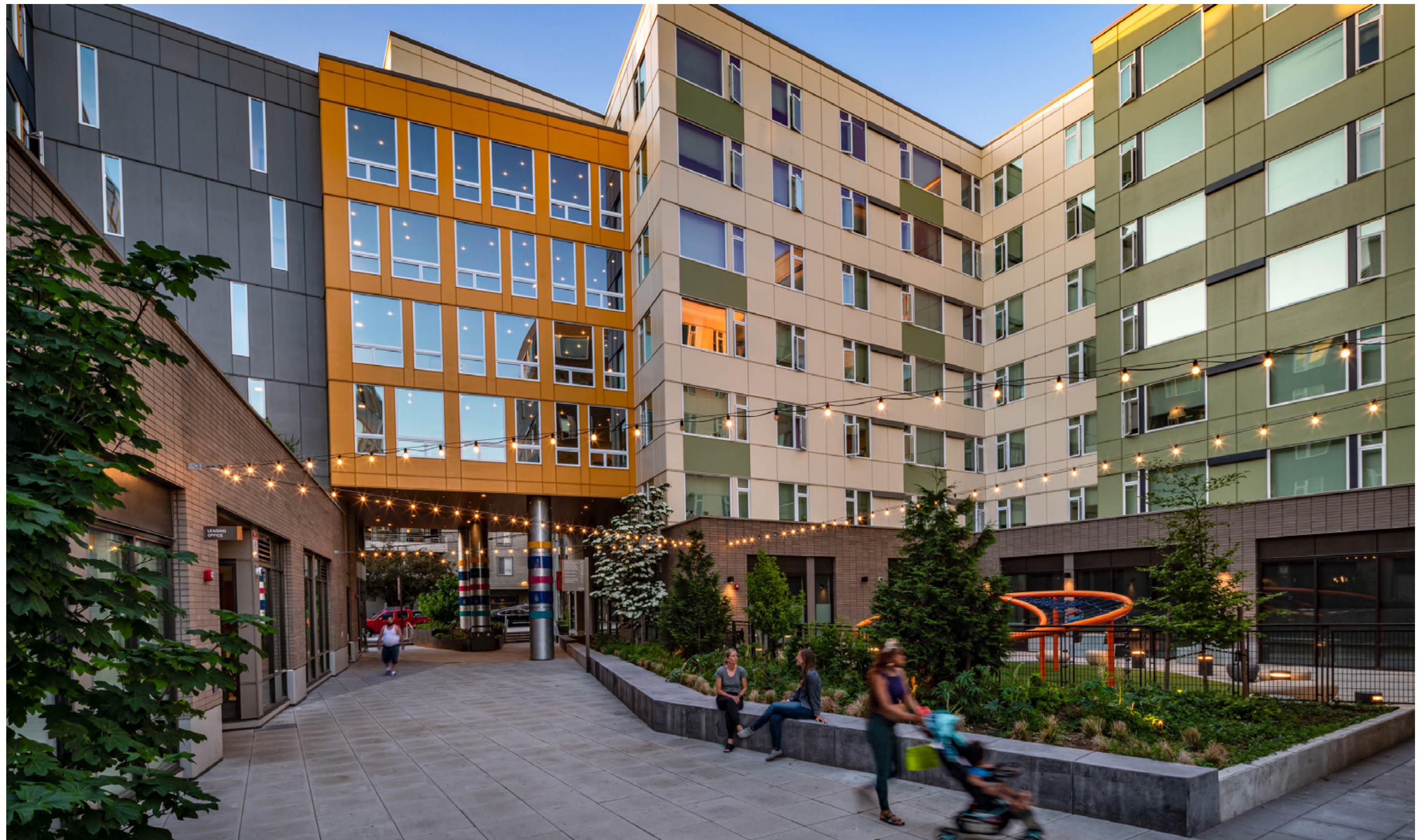
Native Vine Maple/ Acer circinatum , Western Red Cedar/ Thuja plicata , and Western Dogwood/ Cornus nuttallii frame the courtyard and have a significant amount of soil volume and depth created by the angled seat wall. This urban forest in miniature provides important urban habitat to a variety of species and represents a real connection for the residents to nature.
