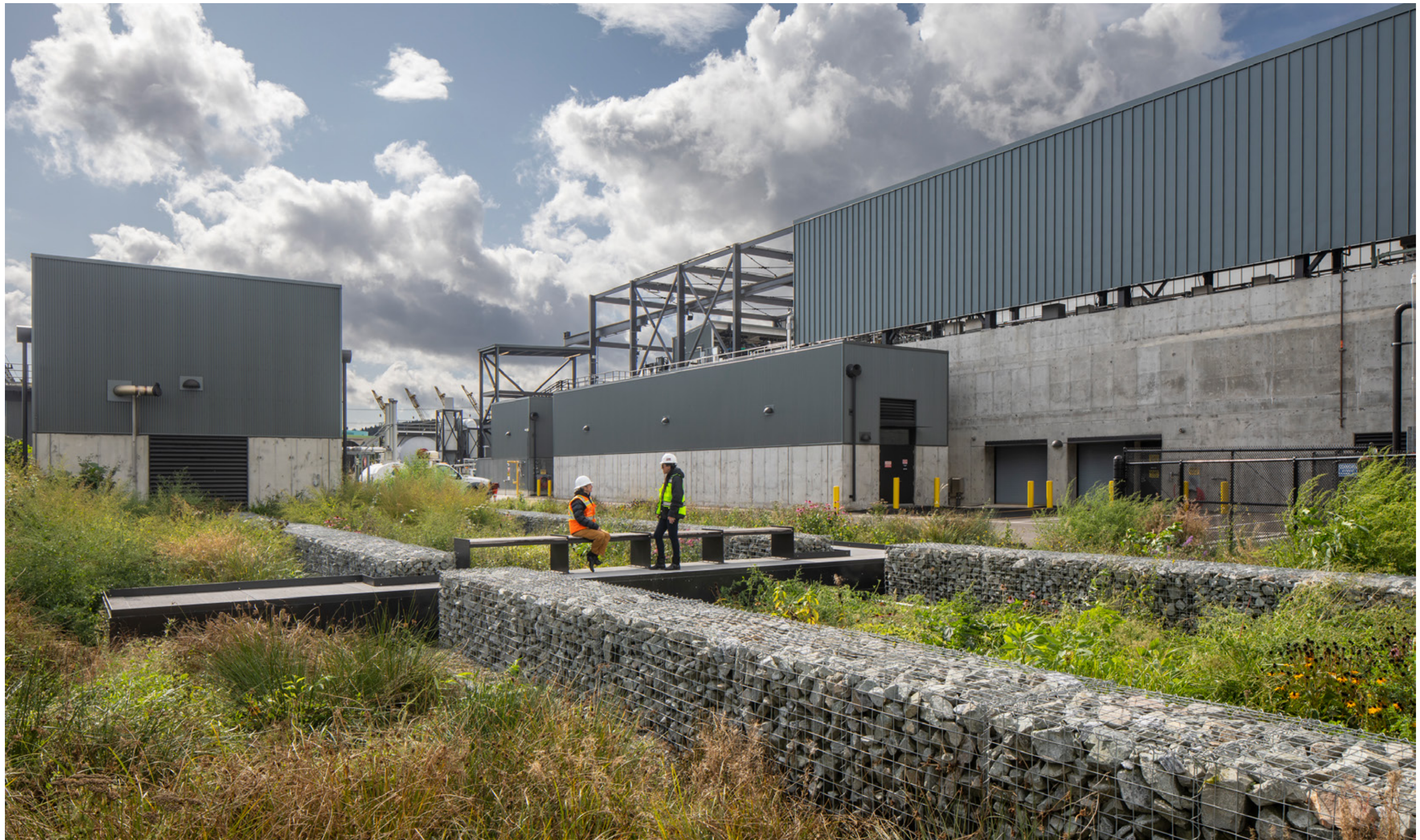
Green stormwater infrastructure performs alongside the mechanical systems by processing all rainwater that falls onsite. The large bioretention facility is visible from the street and accessible to educational tours, demonstrating its process out in the open.
