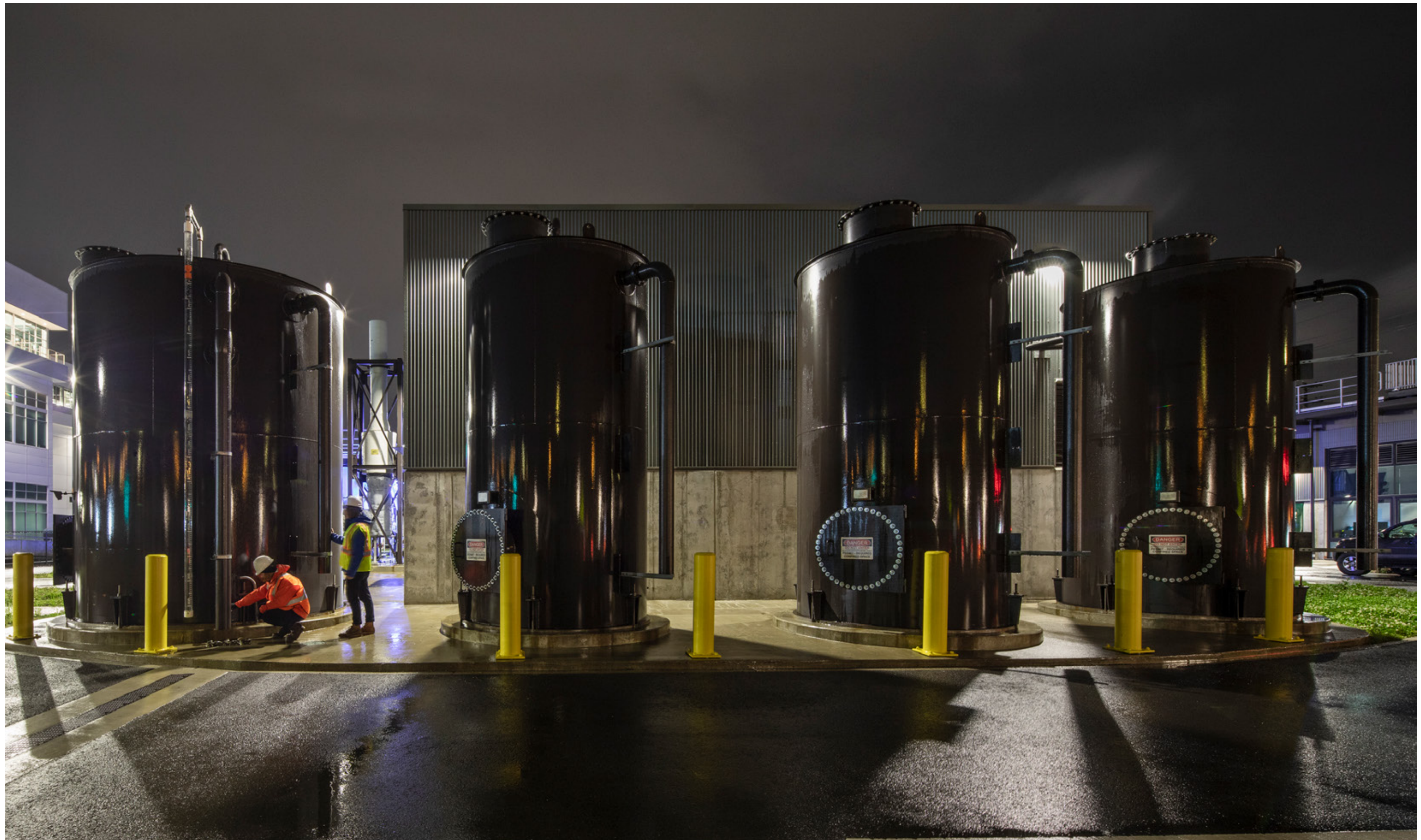
Rain-capturing cisterns hold a combined volume 50,000 gallons and provide about 30% of the site's irrigation, as well as stormwater detention.
