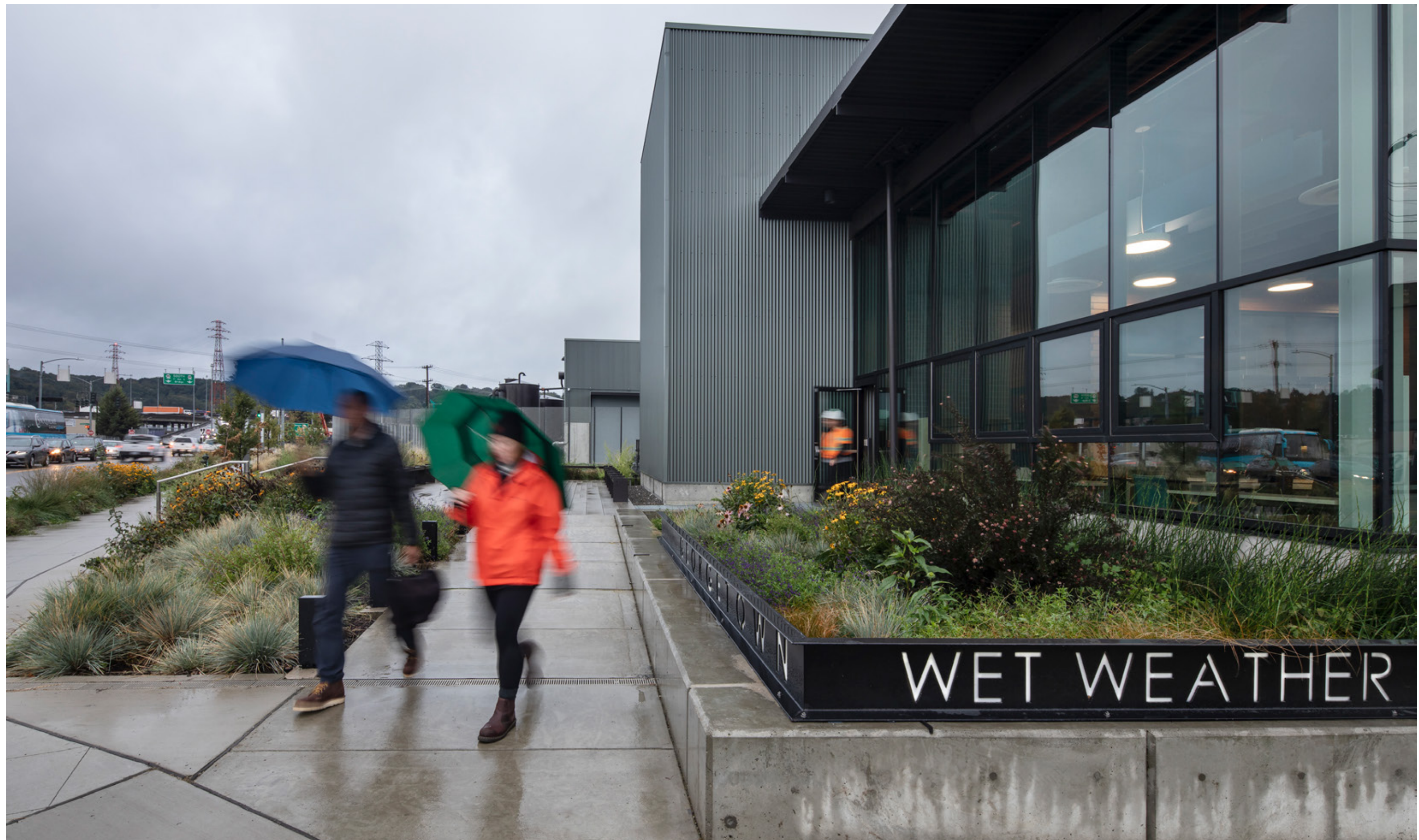
The scale of public and private spaces are balanced along the community edges of the station. The pedestrian entry at 4th Avenue South and South Michigan Street offers a community plaza and public entry to the facility's maintenance and operations building that doubles as community meeting space.
