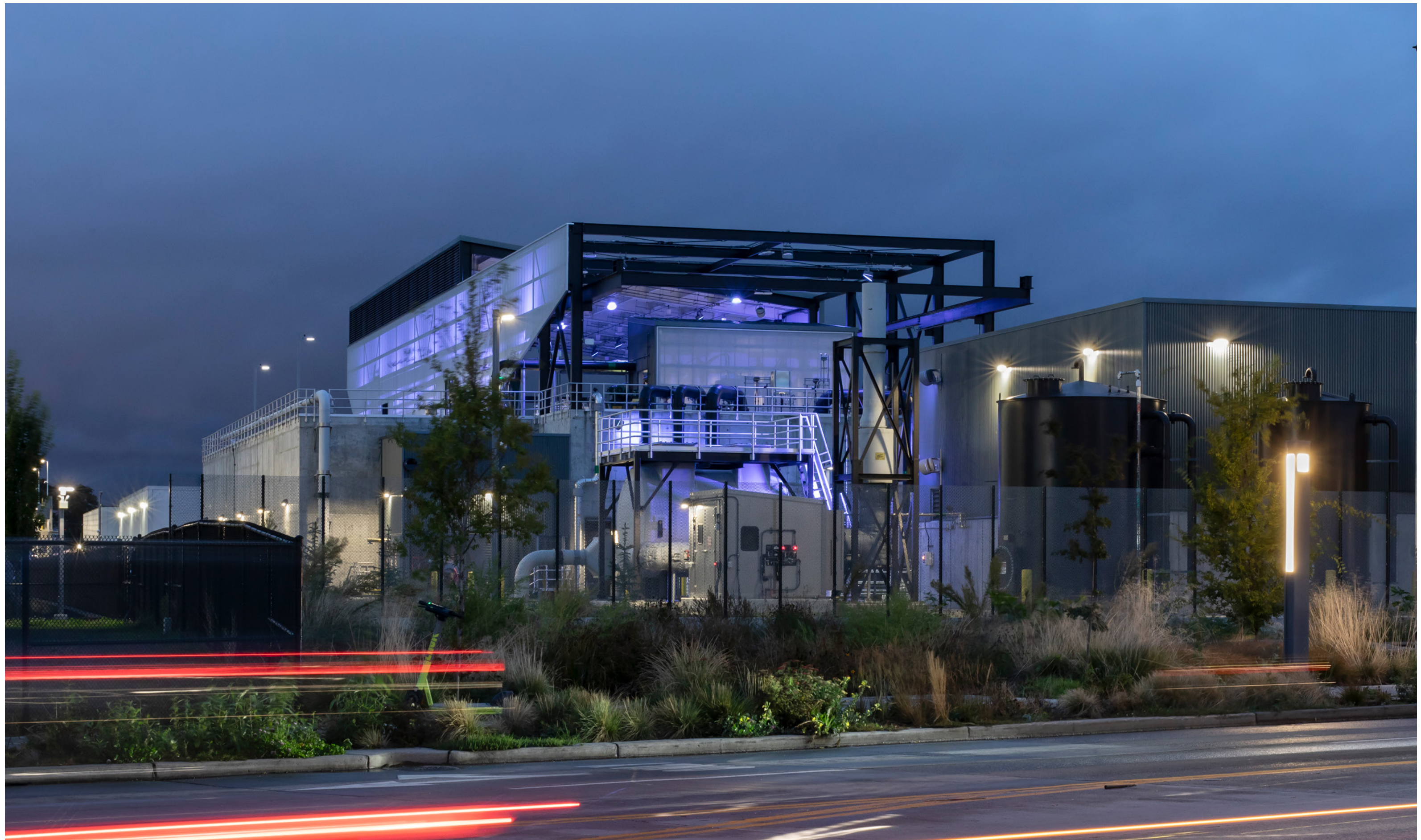
The “Theater of a Storm” art installation indicates and tracks treatment stages with a sequence of lights when the station is operating. The series and duration is always dynamically changing, demonstrating to the community that something is happening at the facility. On the rainiest days the facility will be luminous and working toward improving the health of the Duwamish River.
