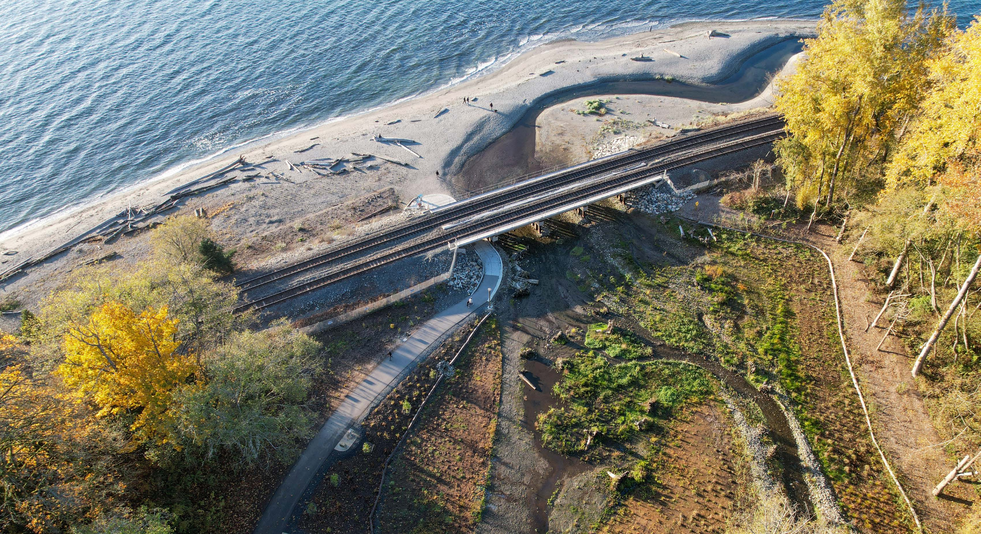
The restored estuary and lower creek freshwater habitats reintroduce shoreline coastal ecosystem processes including creek dynamic meandering, coastal wave influences on sediment transport and deposition, salt and freshwater development in brackish waters, and accumulation of detritus and wood.
