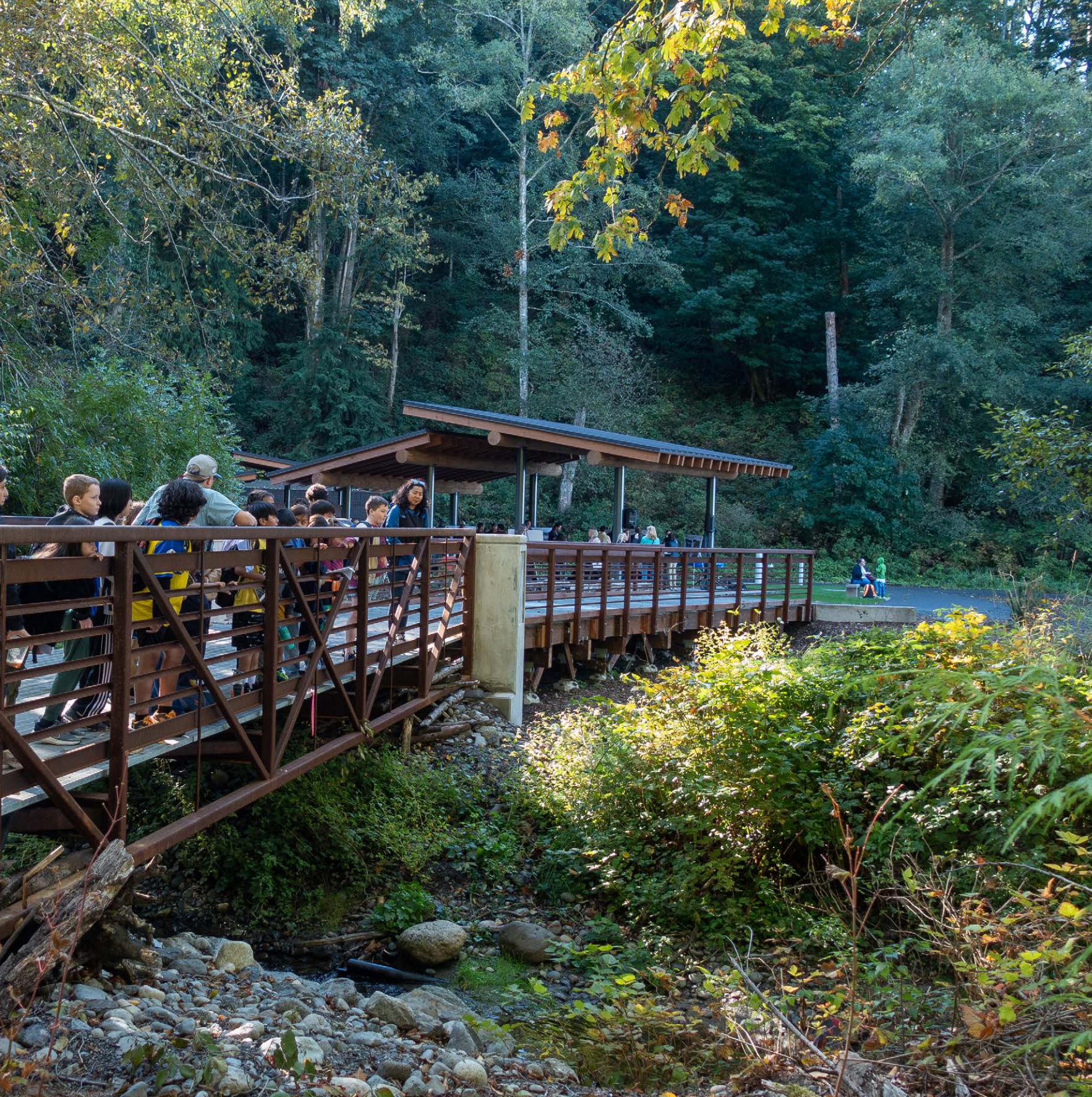
A new concrete and weathering steel pedestrian bridge traverses Lunds Gulch Creek to connect the upper and lower sections of the park and provide views of the salmon-bearing creek. Salvaged trees are used as large woody material and habitat snags throughout the creek and estuary to improve fish habitat.
