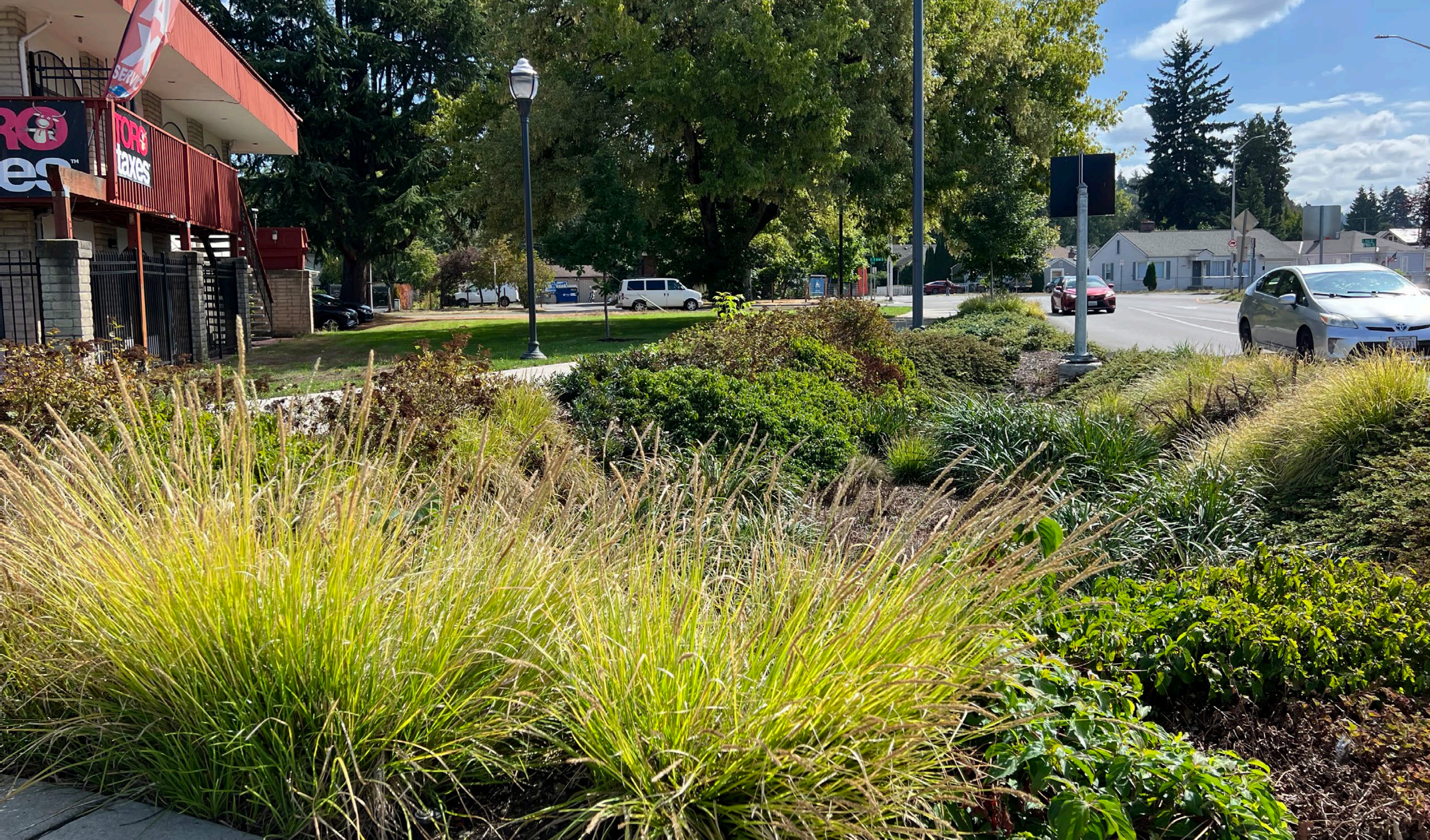
Large planted stormwater raingardens infiltrate runoff from the new roundabout and sidewalk connections as well as soften the expanse of pavement for neighboring businesses and residents.
