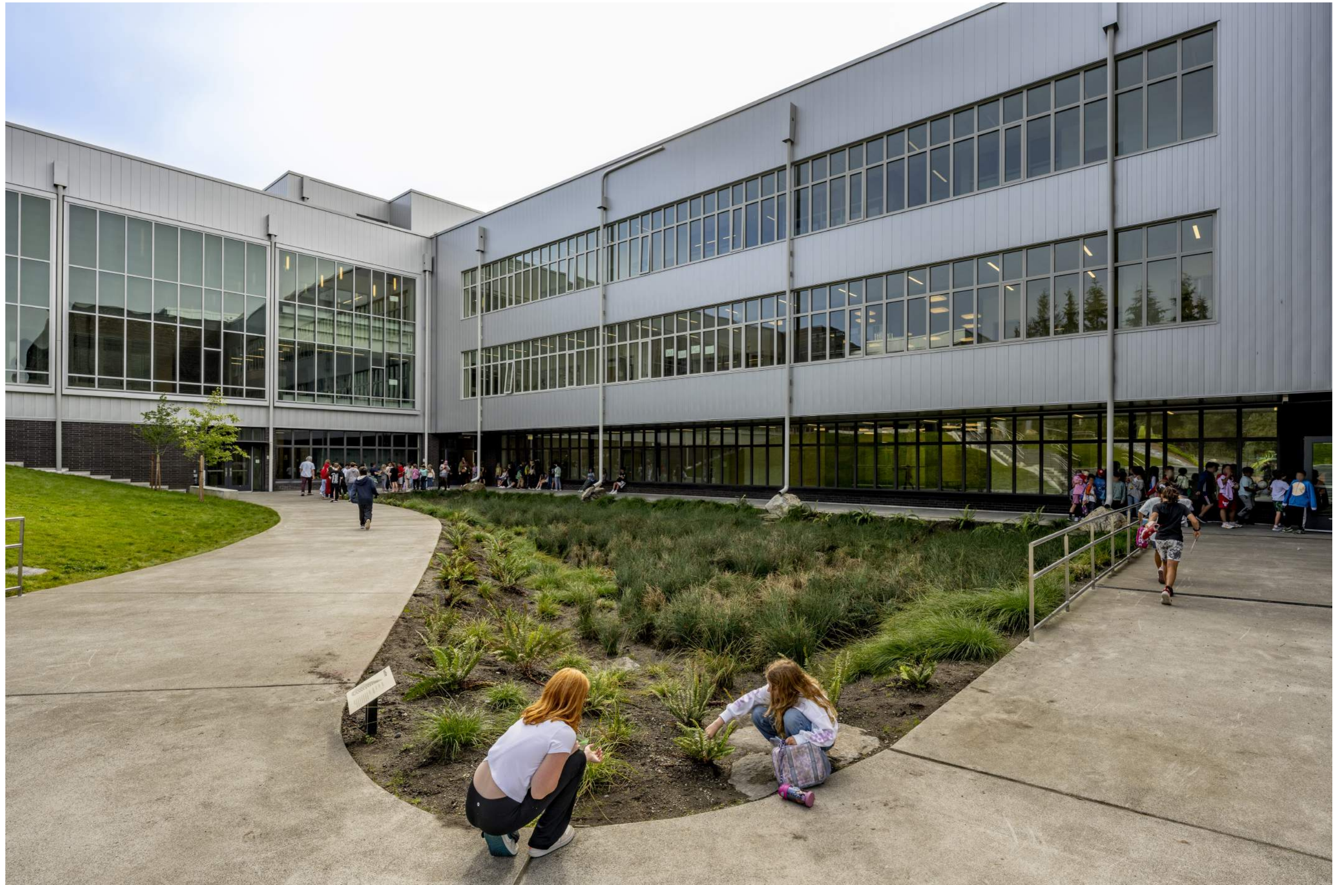
A bioretention cell in the classroom courtyard is part of the daily passage of students. Six bioretention cells in total are integrated throughout the school site, cleansing stormwater and slowing its release into the Piper's Creek watershed.
