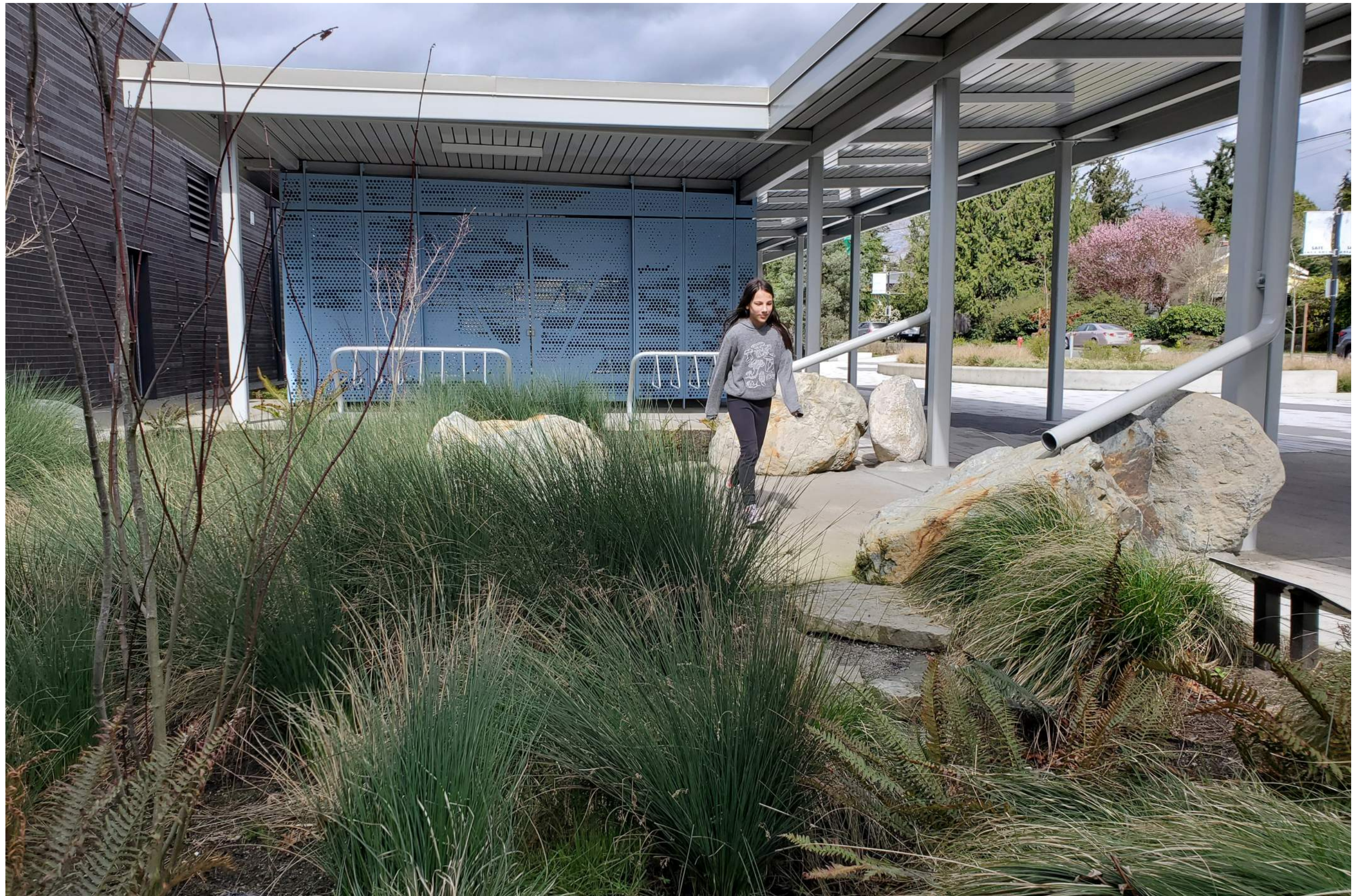
In a small courtyard adjacent to the bicycle parking enclosure, a small bioretention cell provides a learning opportunity as students arrive at school. Native species, educational signage and swooped downspouts highlight the connections between stormwater and natural
