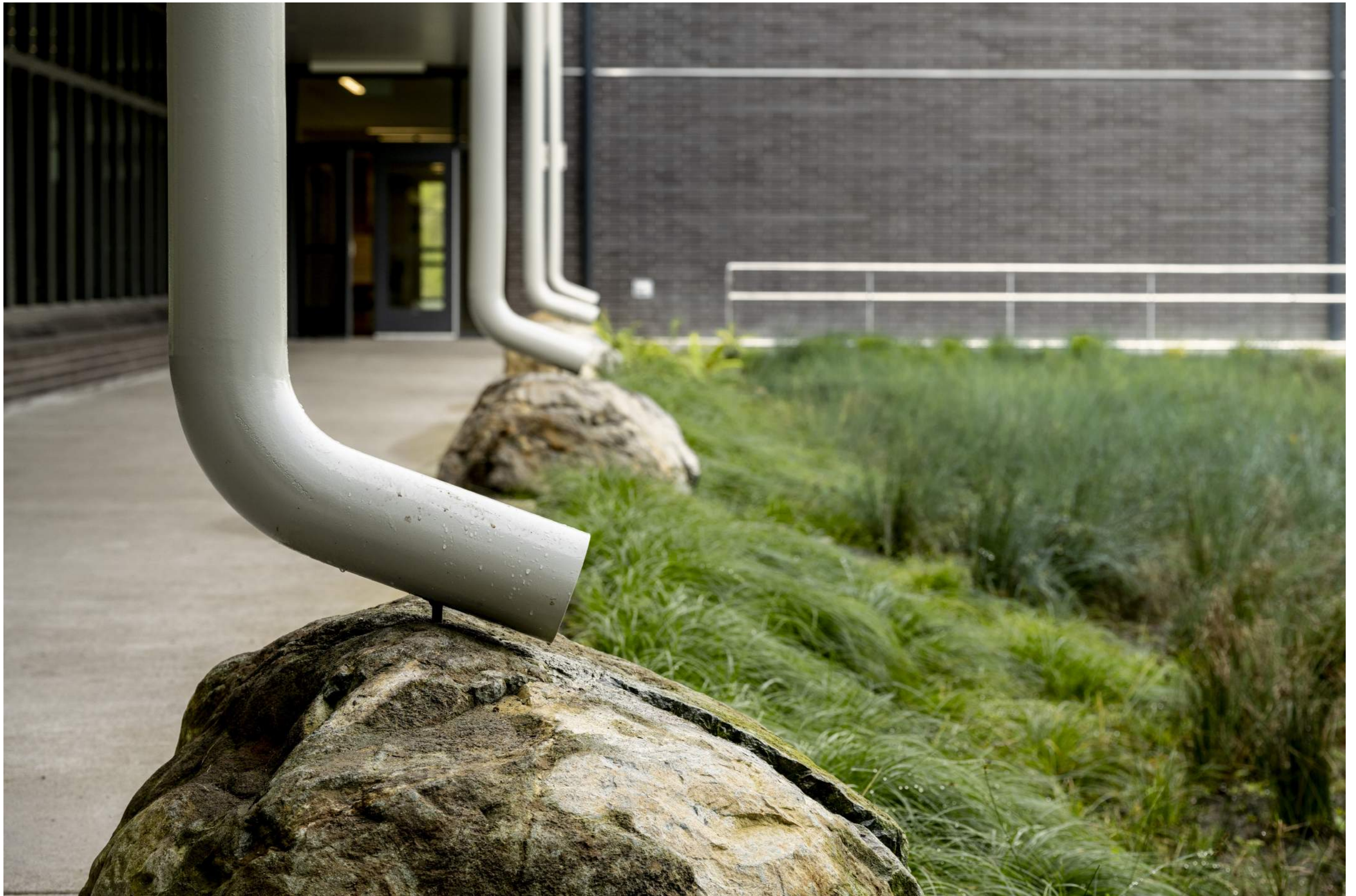
The design team developed custom details to celebrate the flow of stormwater from roof to bioretention cell. The boulders sit above natural stone steps, dissipating and displaying water flows from the covered walkway.
