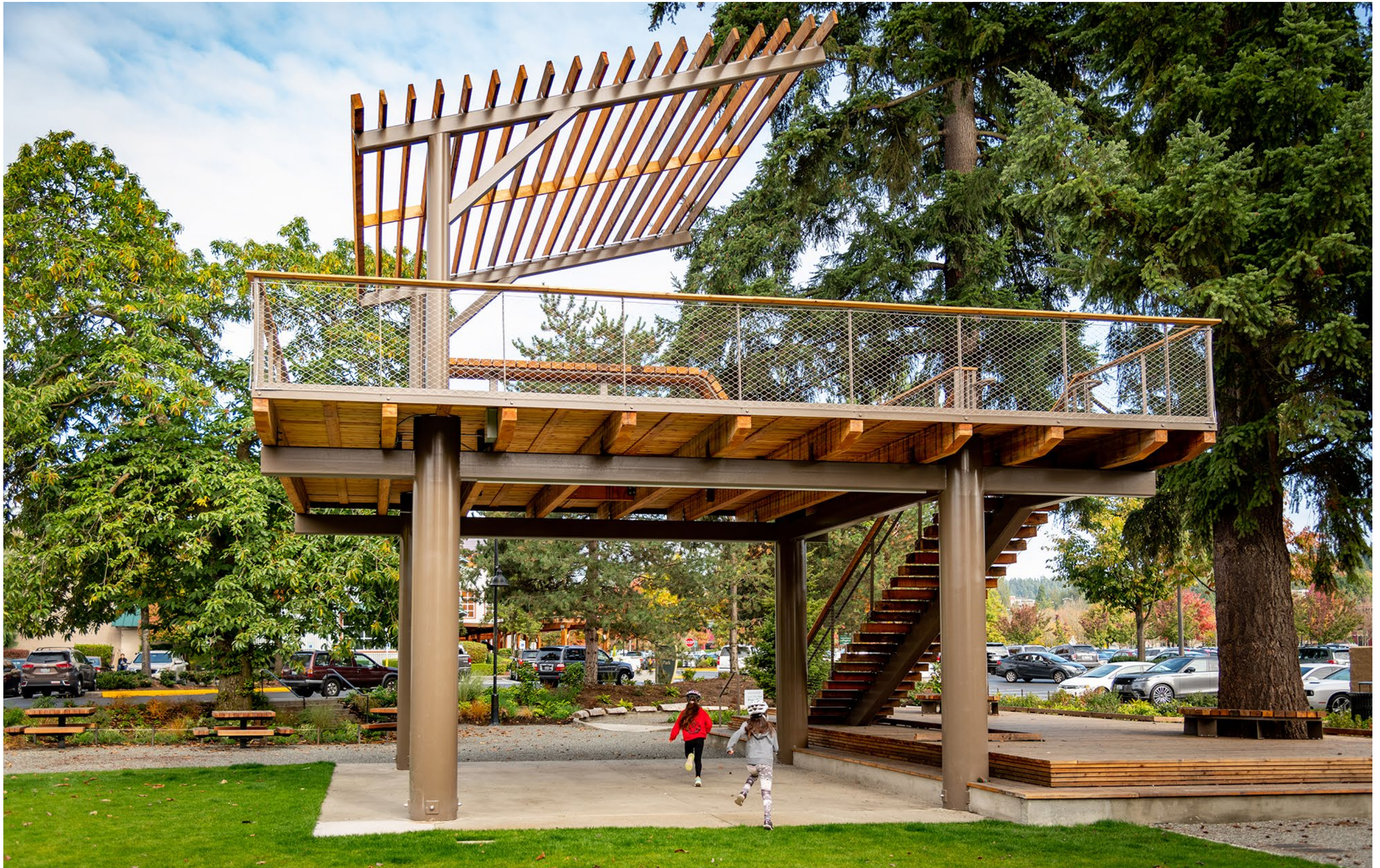
At the treehouse base, a lower deck visually anchors the structure with the site and provides an accessible place to more closely engage with the trees, while protecting their root systems.
