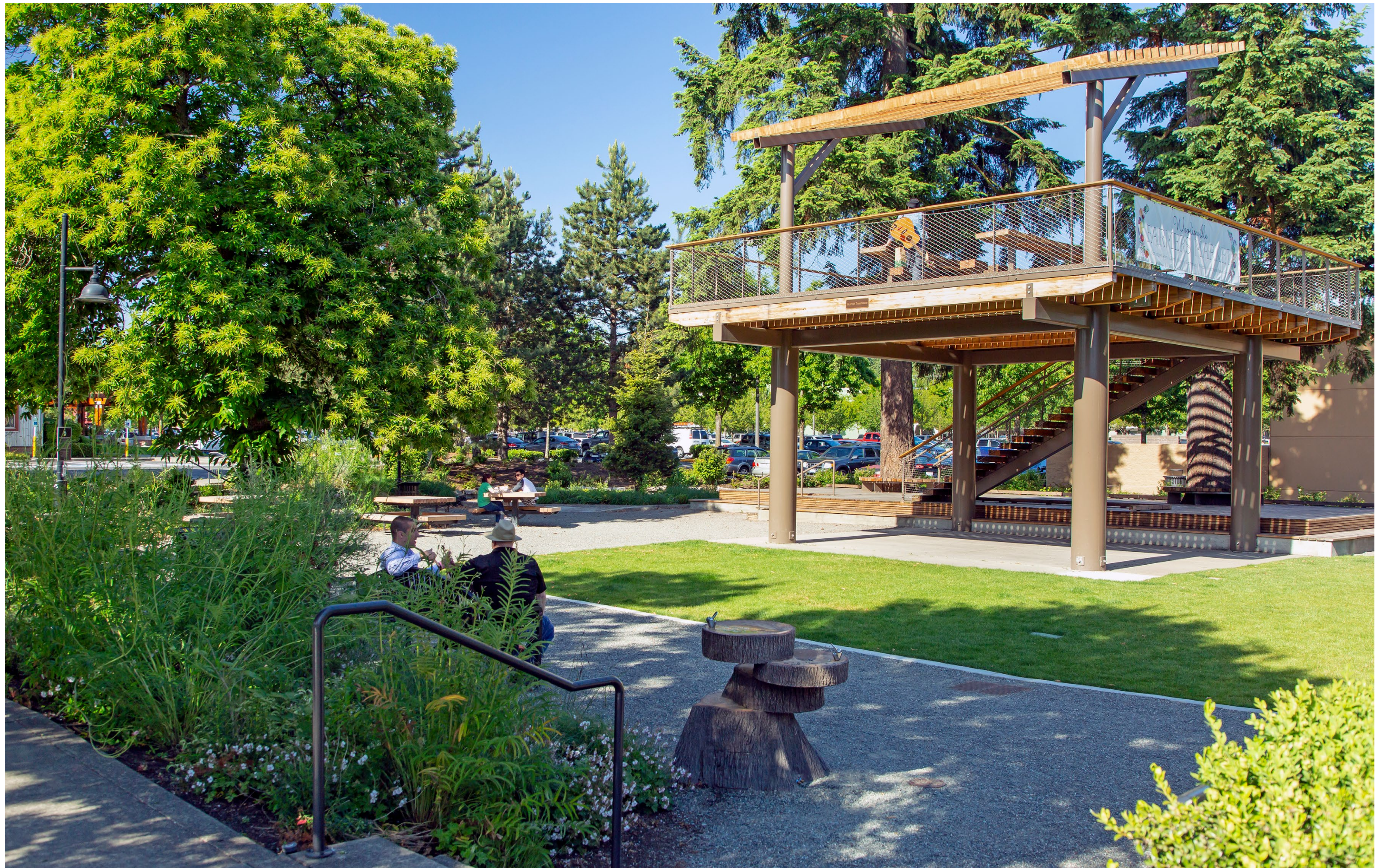
Steel supports wrap the original columns to provide structural integrity and the vertical clearance needed to host events below in a weather protected space.
