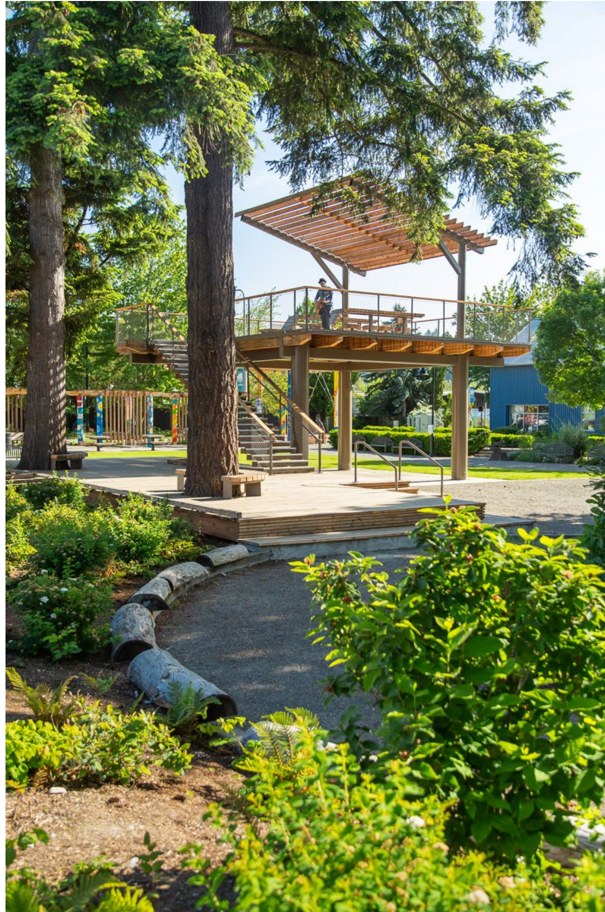
The wood salvaged from the park's former gazebo and trellis structures was crafted into the treehouse stair treads and custom seating as well as the two curved benches that wrap the Douglas firs at the lower deck.
