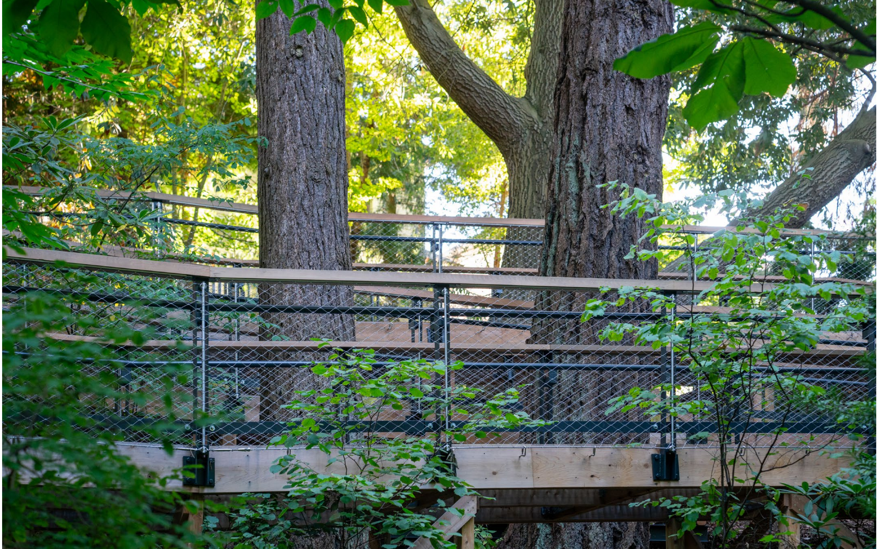
The materials chosen for the boardwalk were carefully selected to complement the natural surroundings so the boardwalk could blend into the canopy over time.
