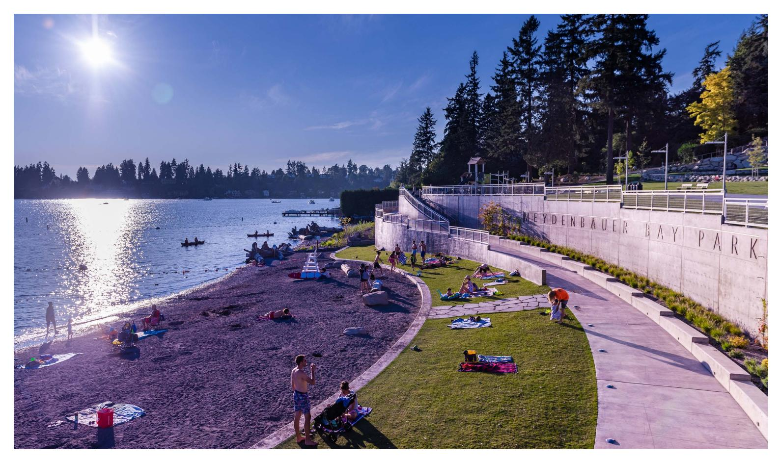
Complex concrete retaining wall design—adorned with the park's name, vines, and grasses—and extensive site grading offer a dramatic backdrop. The walls cut into the steep hillside to provide a flat, sandy place to soak up the sun.
