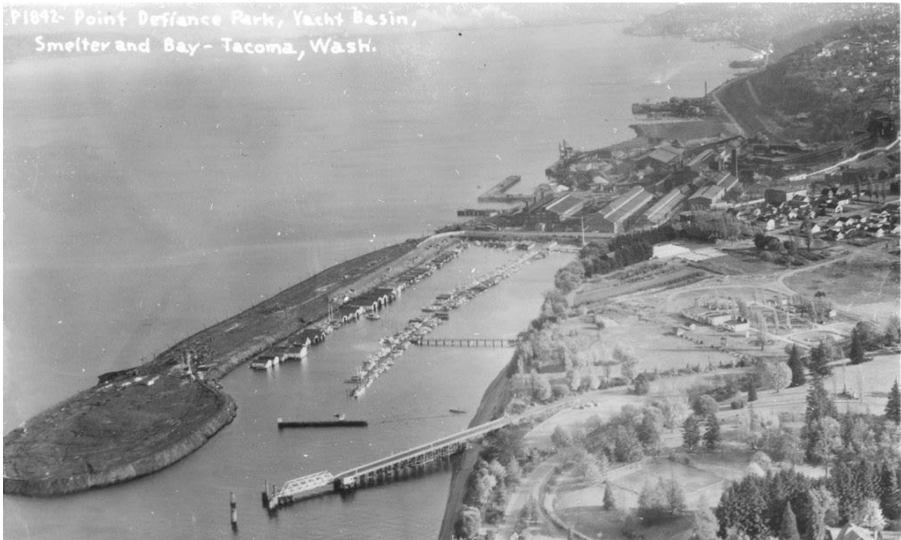
The project site was home to the ASARCO copper smelter for over 70 years, and the community saw its 571-foot smokestack as a symbol for jobs and an ominous source of widespread pollution.
