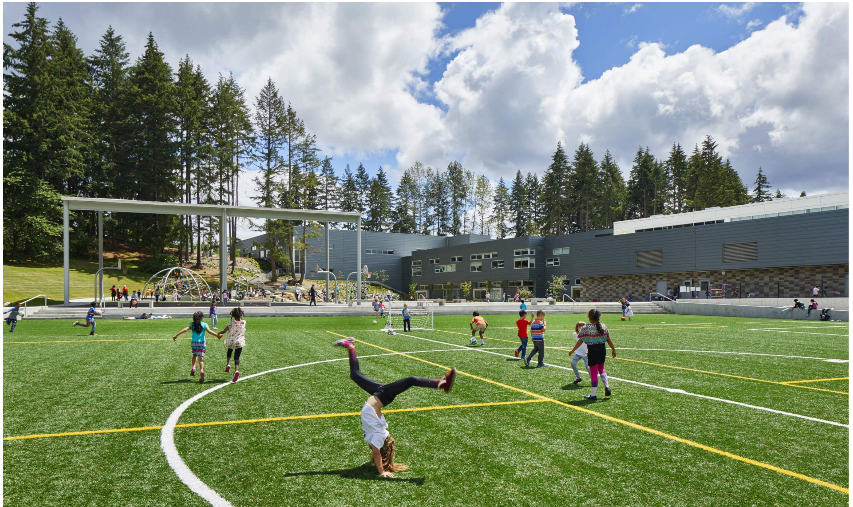
Bennet Elementary's stepped configuration allowed it to be carefully inserted into the wooded slope, preserving richer views of vegetation. The fields were sited on previously paved, flat portions of the site and use recycled cork as a natural infill product.
