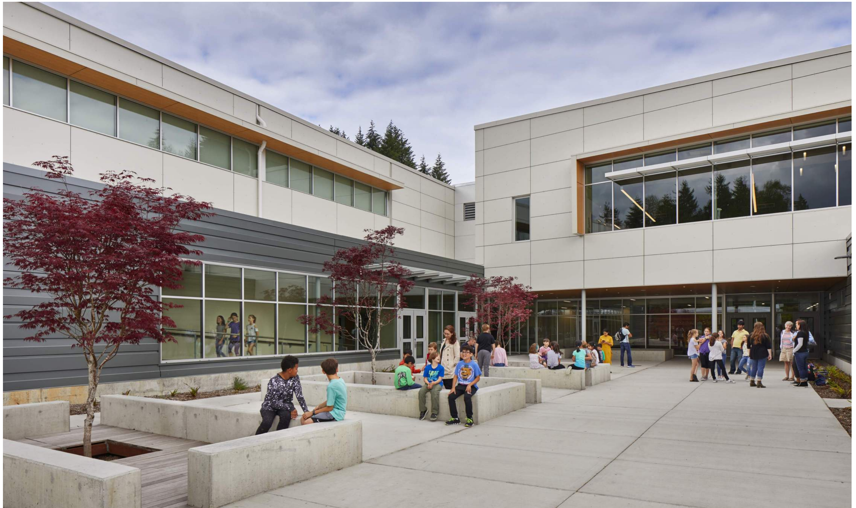
The entrance to Bennett Elementary emphasizes interaction between students, teachers, parents and community members with these concrete 'council rings'.
