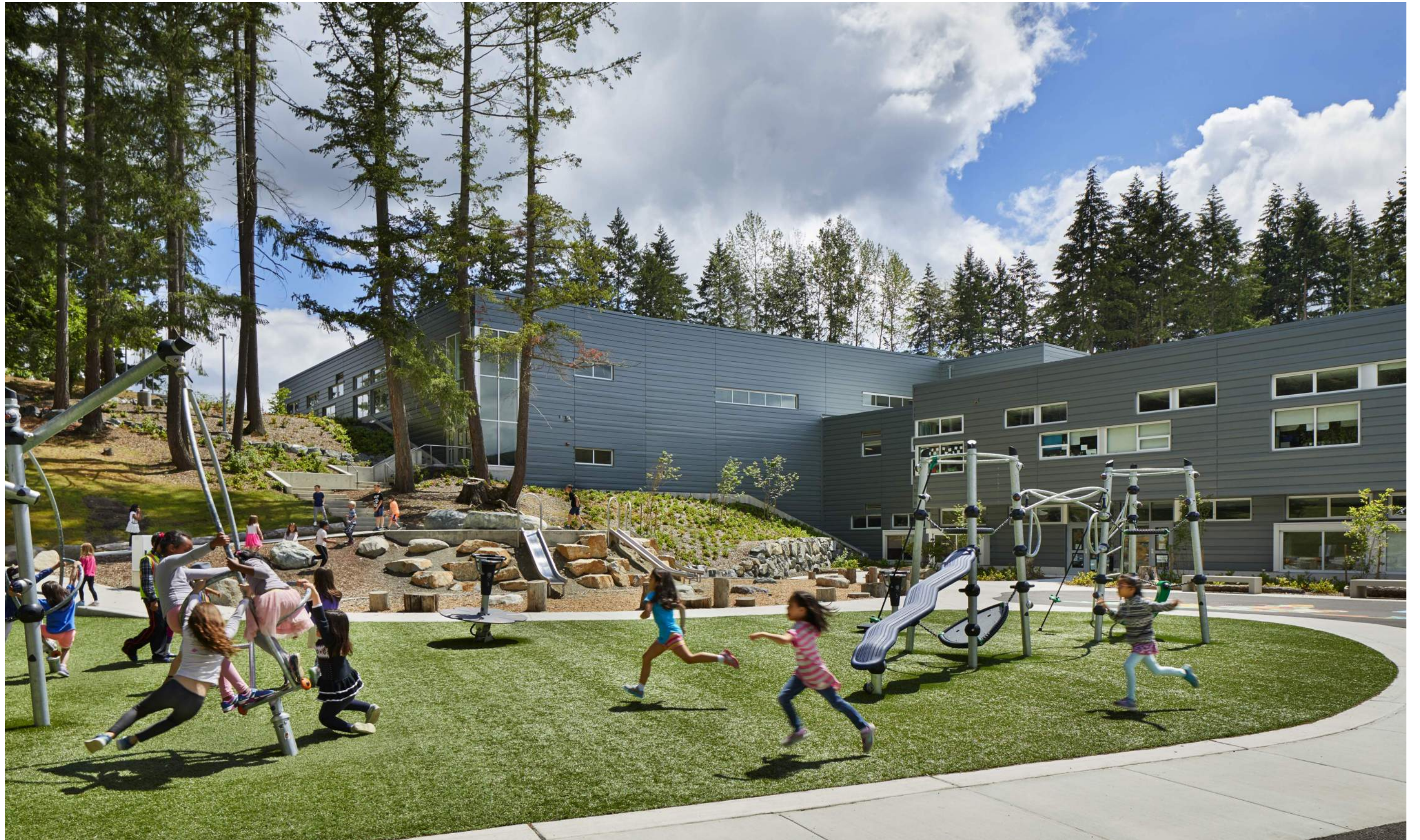
Boulders unearthed during construction are re-used in a natural play area, creating a perfect transition between the wooded slope and the cork-filled, synthetic play areas, and offering children choice in how they play.
