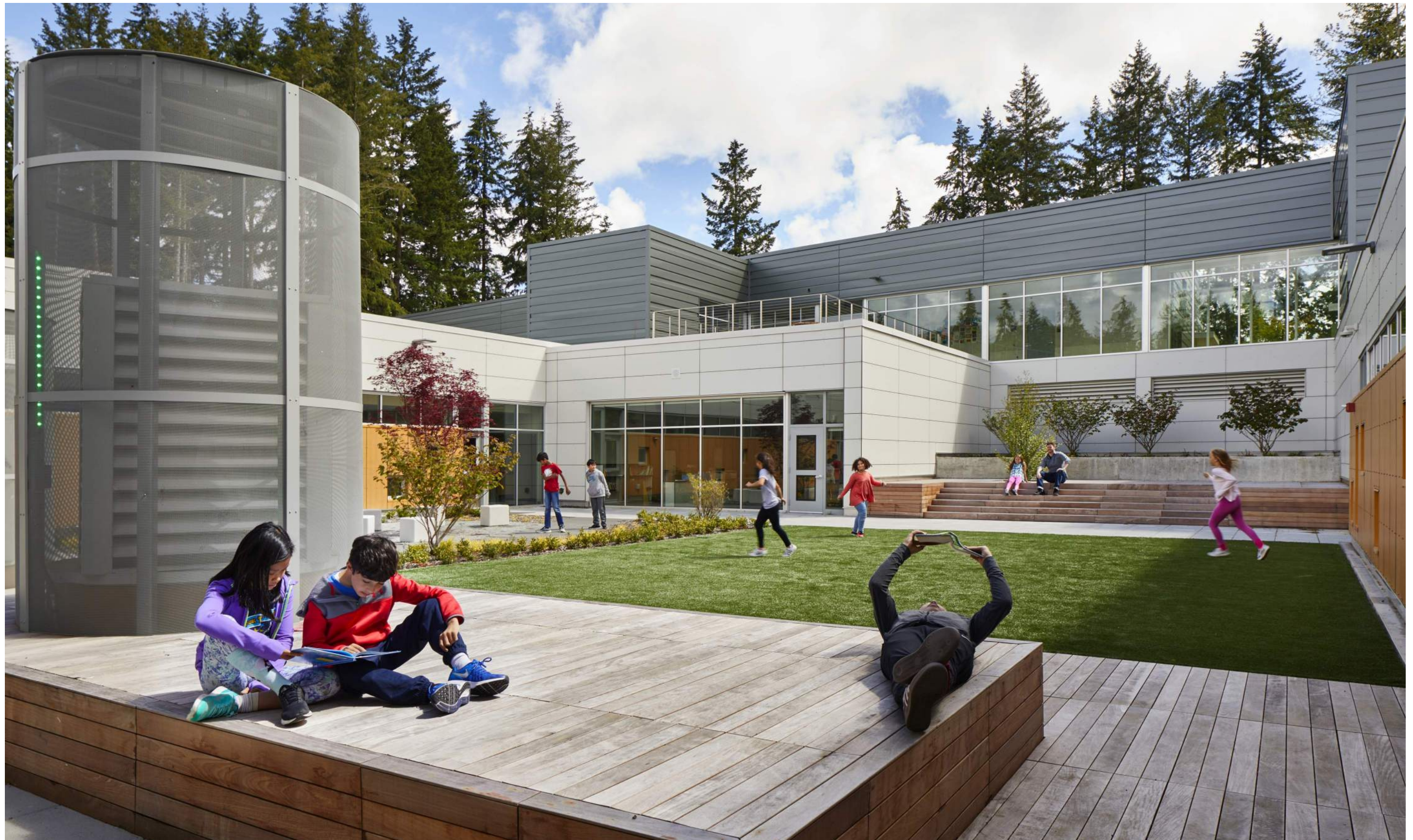
An interior courtyard with a synthetic play lawn allows natural light to flood multiple stories, and resolves the difficult grade changes.
