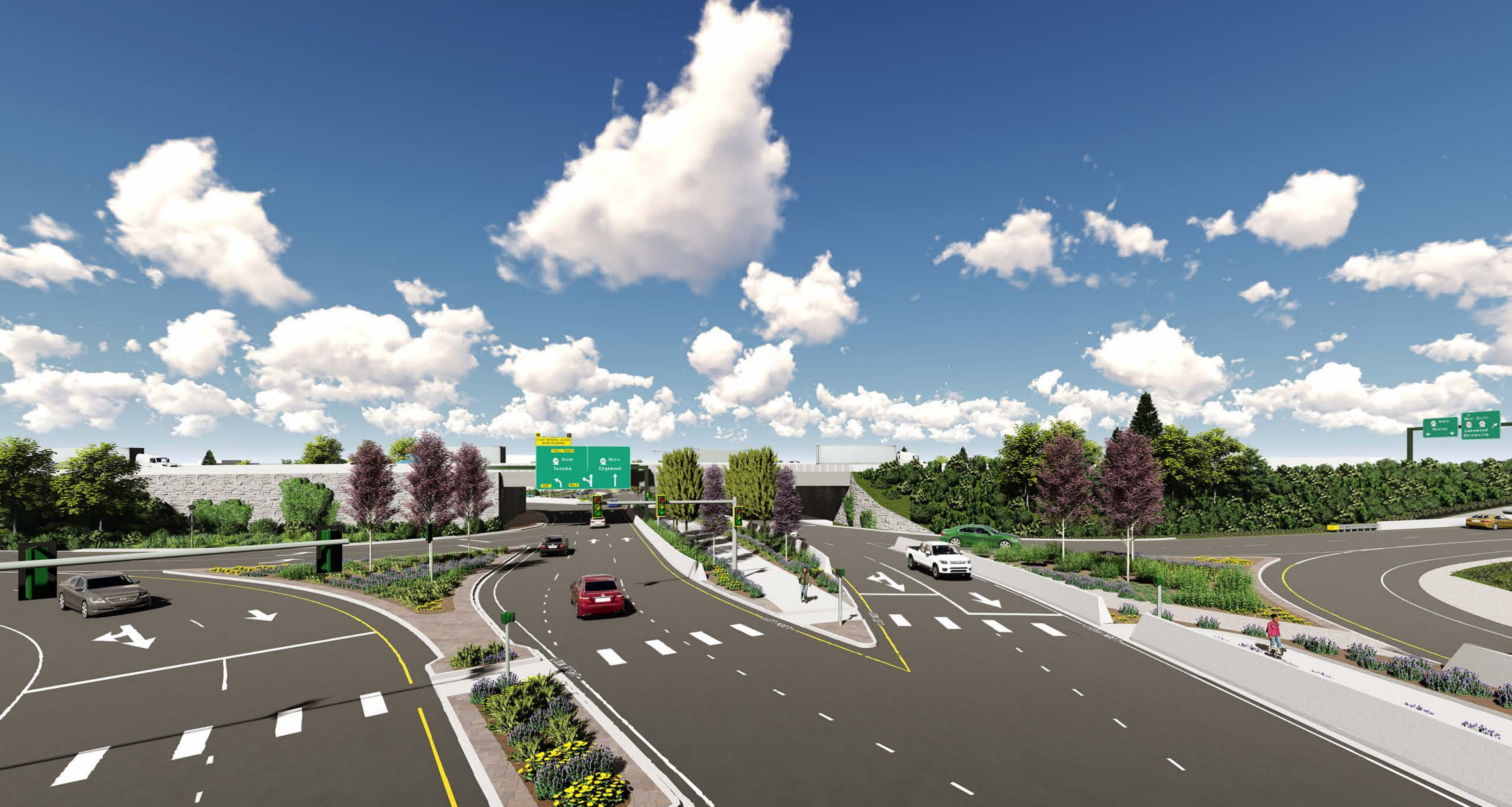
DIVERGING DIAMOND INTERCHANGE | Rendering of the SR 167 Overpass and N Meridian Ave Junction: Visual Approaches, Pedestrian Connections, and Street Landscape Treatments.
