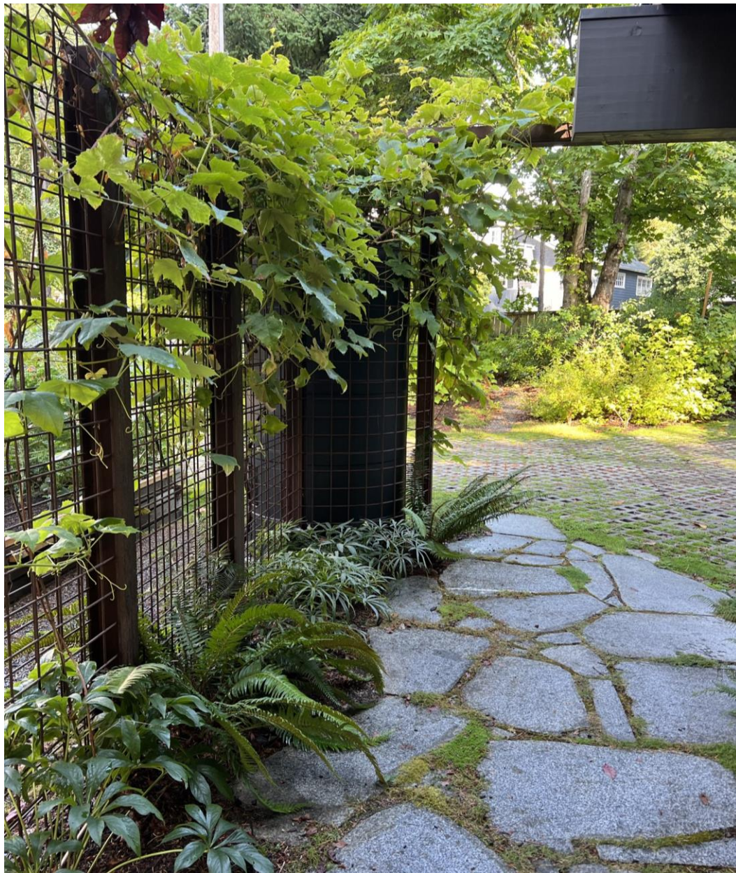
At the site entry, above-ground rainwater cisterns are filled with runoff from the carport roof. Cisterns are wrapped in steel mesh and planted with grapes. The veggie garden is to the left of the mesh fence, along the quiet lane. A community berry bramble can be seen across the driveway. Local Cascade granite with planted joints was used for pedestrian paving; driveway is Turfstone, with openings planted with drought tolerant creeping plants.
