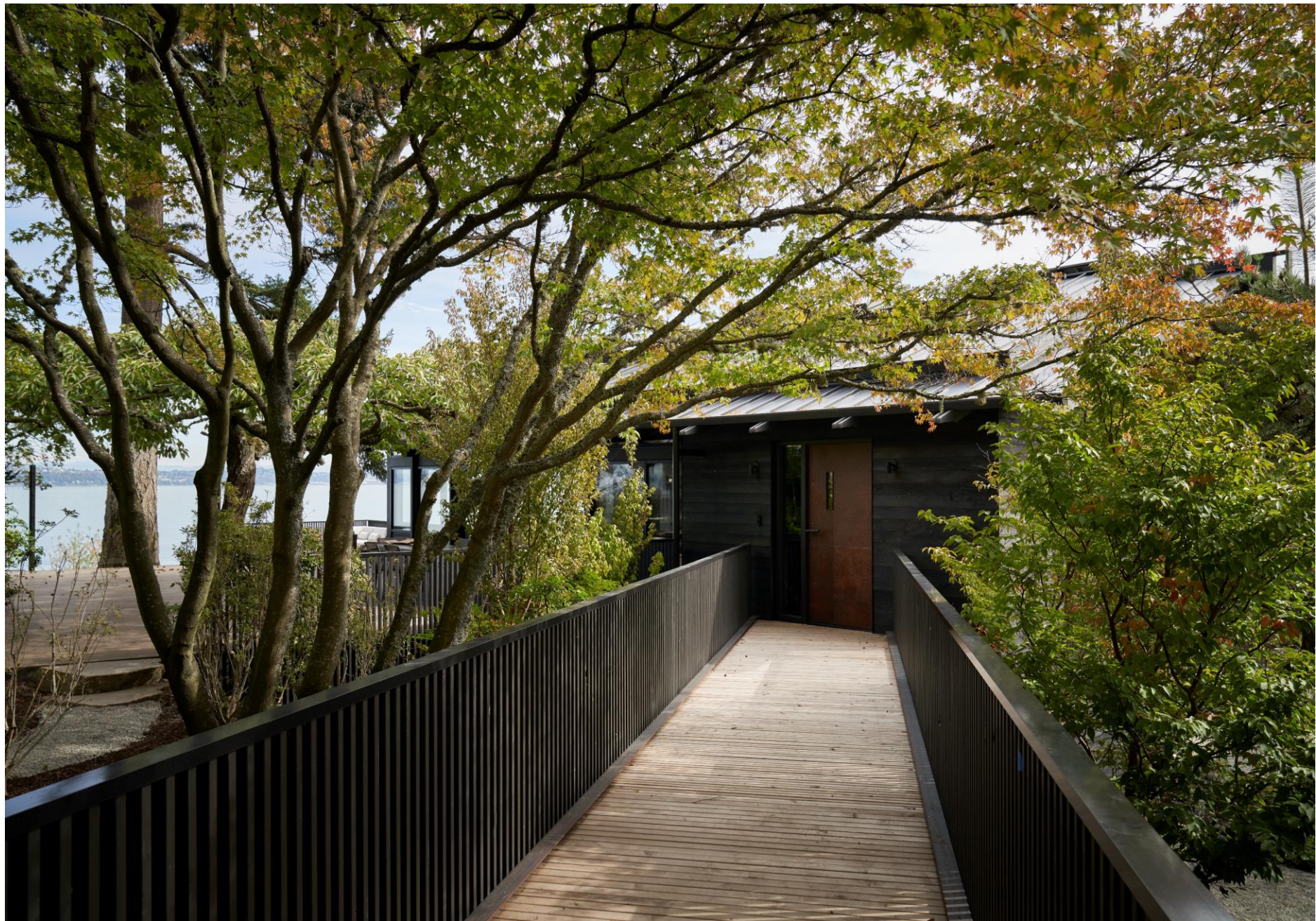
A new elevated walkway built of reclaimed wood leads to the new primary entry; the bridge spans over the landscape, minimizing disturbance to tree roots.
