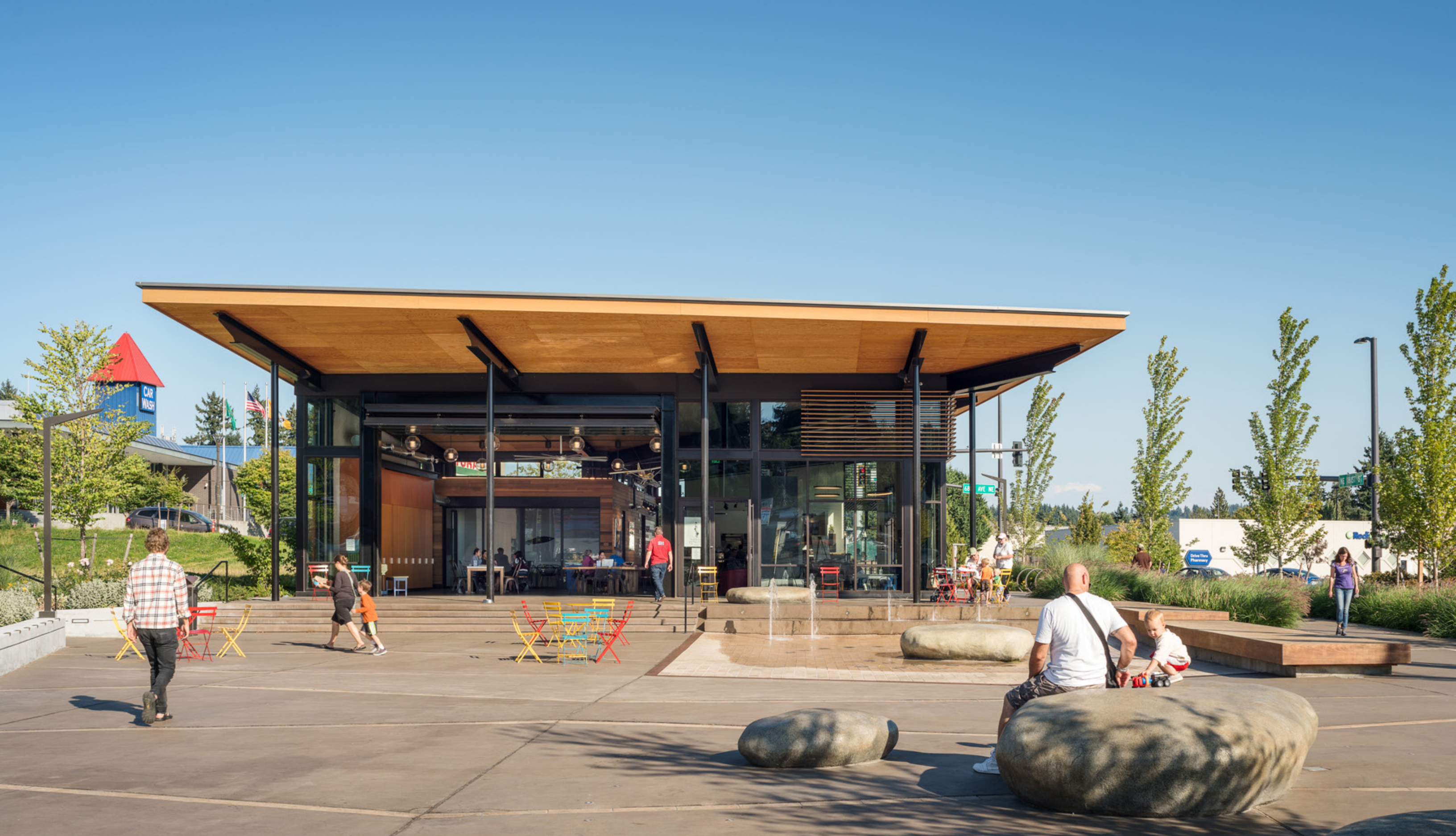
The choreography of the heated rocks and the LED in-grade lights reference the notion of skipping stones at a lake's edge. The heavy timber dock provides seating opportunities to rest and interact with the water feature. The stairs create a porch like, elevated perch, which is a viewing platform into the plaza as well as the potential to become a stage for performances.
