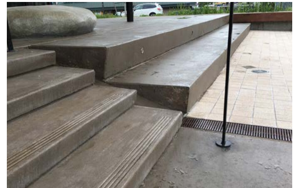
Stair and bleacher runnel interface
