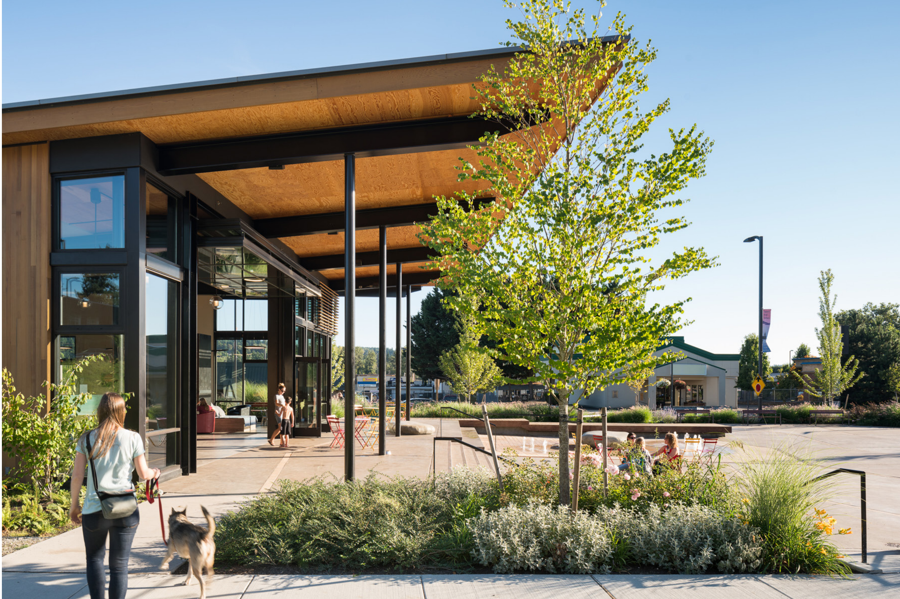
The building's western roof extension provides a weather-protected porch-like area and vantage point into the plaza space. Accessible routes run along the northern and southern edges of the site and both support ADA access to the porch, building entrance and the plaza space.
