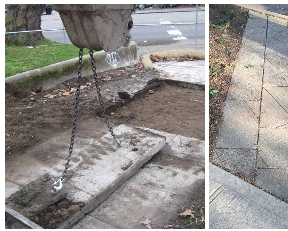
Existing concrete sidewalks crowding the trees were salvaged for reuse. The concrete was sawcut into new largeand small-scale modules and reinstalled onsite to serve as pavers and stair treads.
