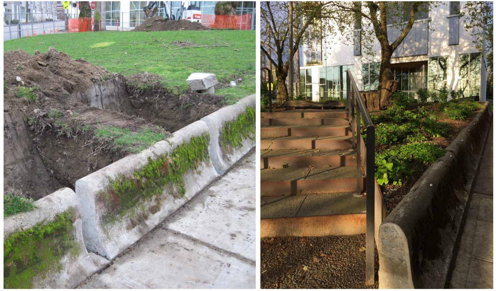
The design preserved the existing raised concrete planter walls but strategically removed two sections enabling barrier-free access into center of the tree canopy. Removed sections were retained onsite as remnants and reinforce the concept of material salvage and reuse.
