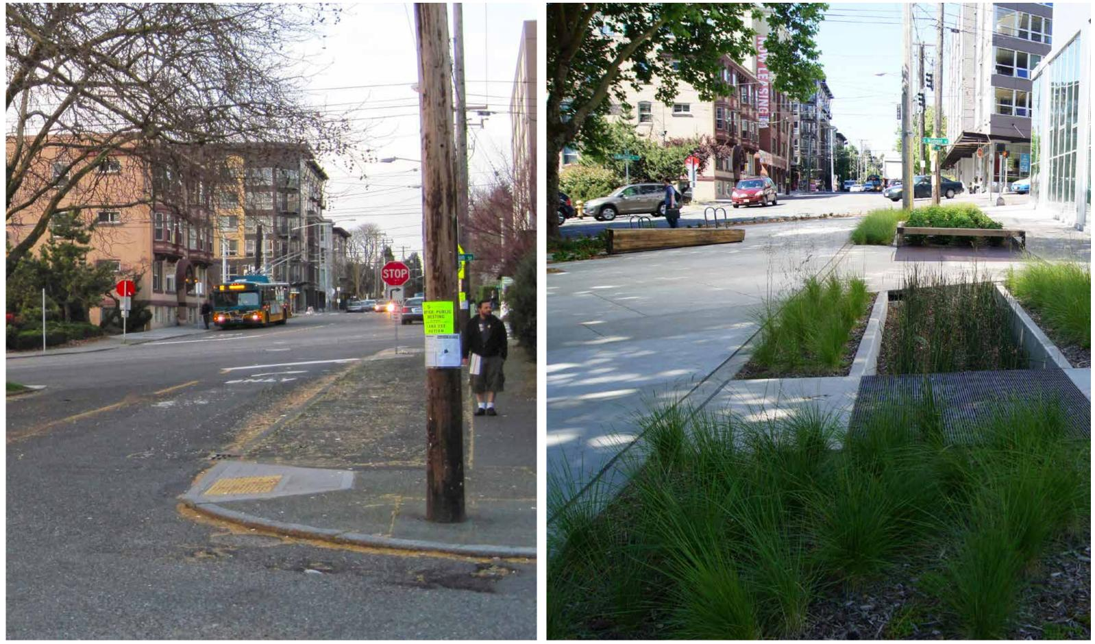
Plantings on 15th Avenue cleanse and filter the site's greywater and stormwater. Species selected for the rain garden and infiltration planter tolerate wide fluctuations in moisture levels. The palette was chosen to make its functions visually intuitive to the public.
