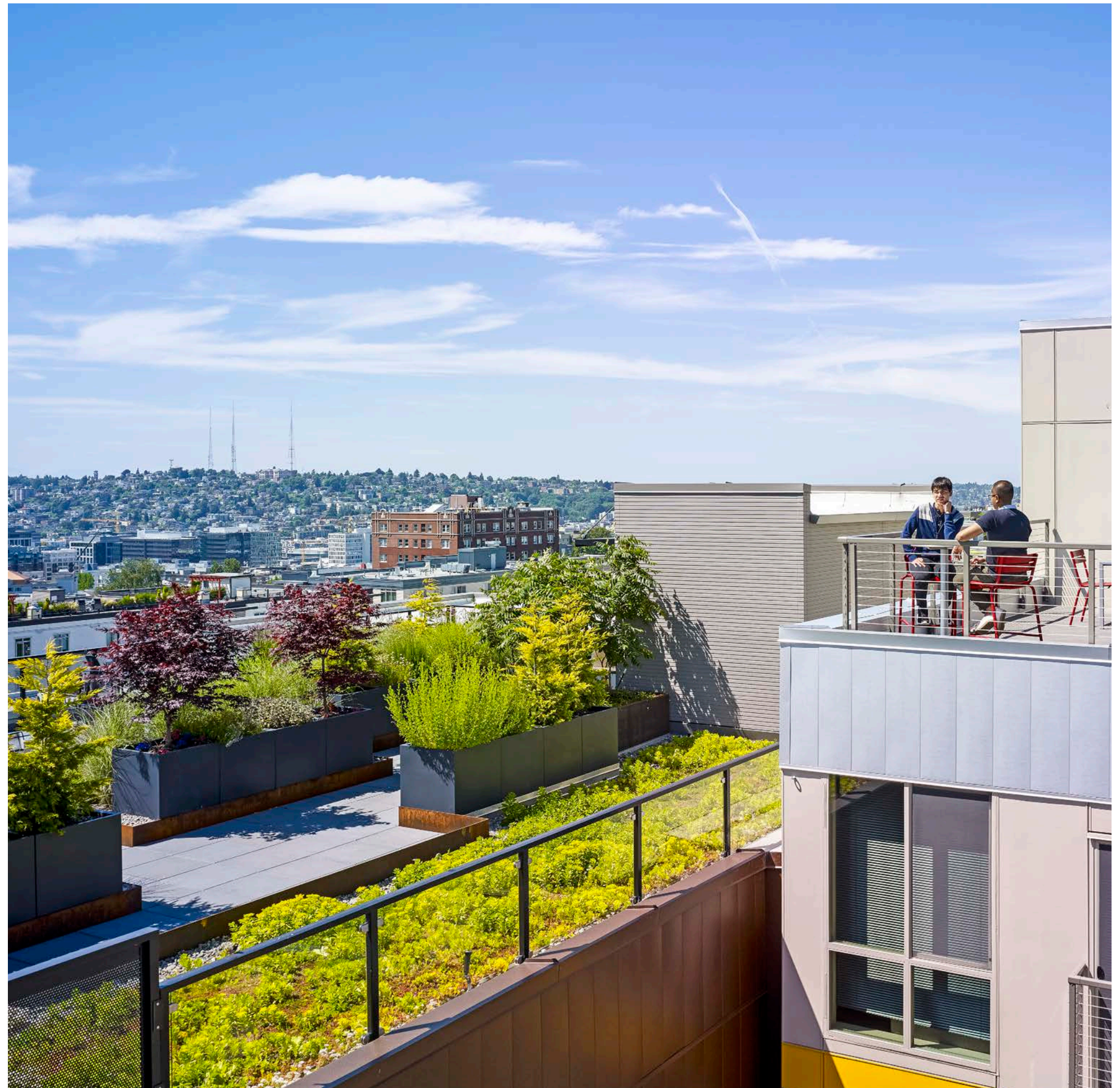
Pike Motorworks' rooftop planters and green roof provide some measure of stormwater mitigation while also visually enhancing rooftop amenity space for the neighboring Cue Apartments.
