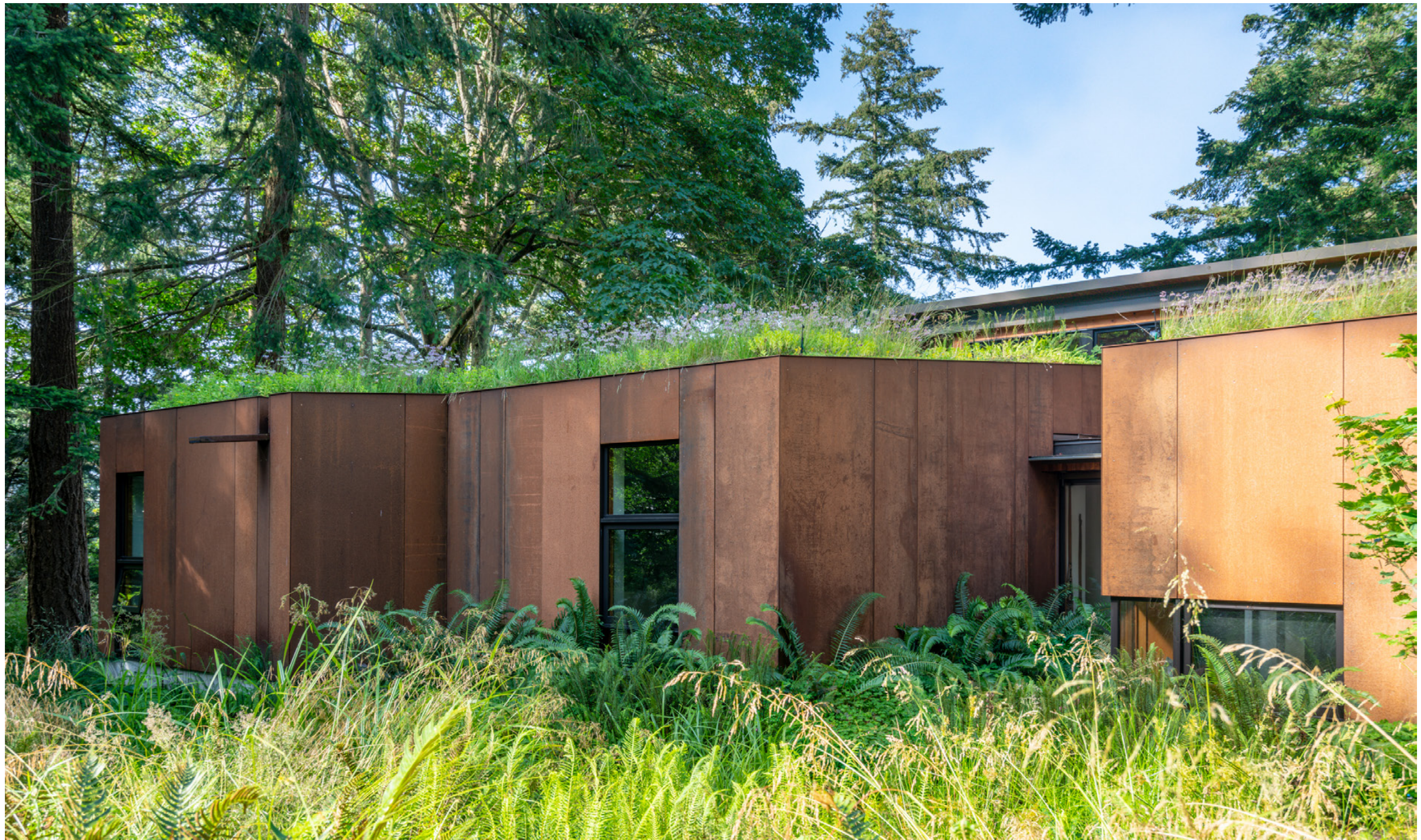
On the forest side of the house, the landscape envelops the steel clad volumes dubbed the “erratics.” The rain garden collects site and roof runoff and provides a distinctly different experience from the water side.
