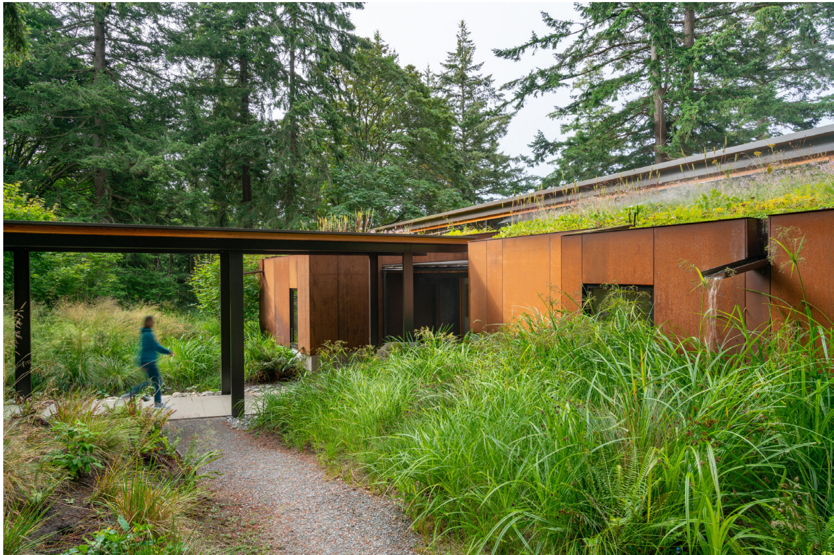
A vegetated roof integrates the main home within its forested setting and provides an entry experience of immersion with views of the rain garden and the sound of water falling from the scuppers.
